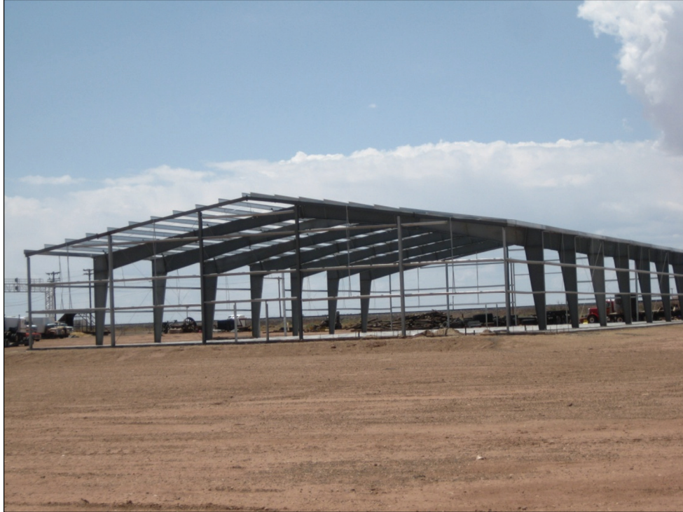
Figure 10-1: Photograph of Metal Building under Construction
