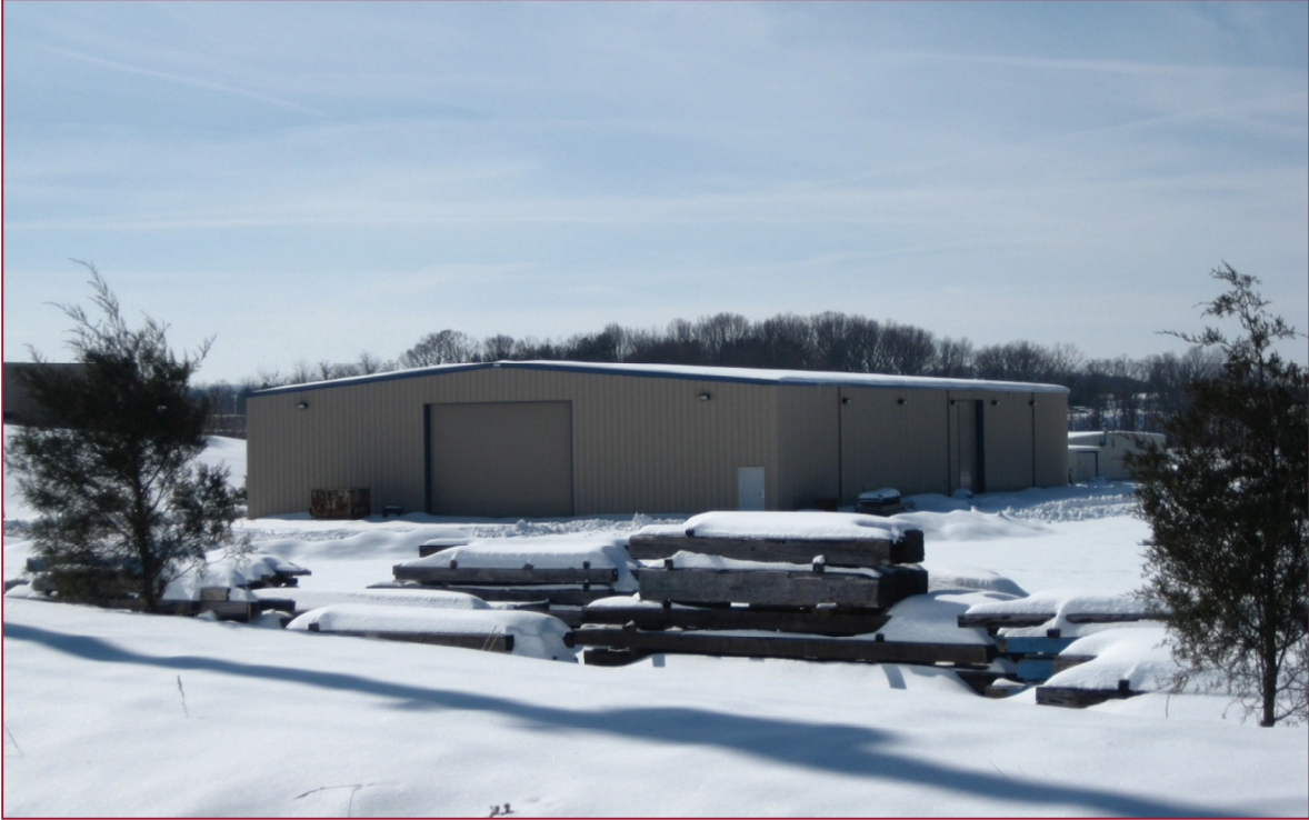
Figure 4-1: Photograph of Exterior of Test Building
