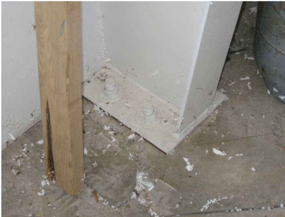
Figure 4-15: Photograph of typical Column Base Connection
