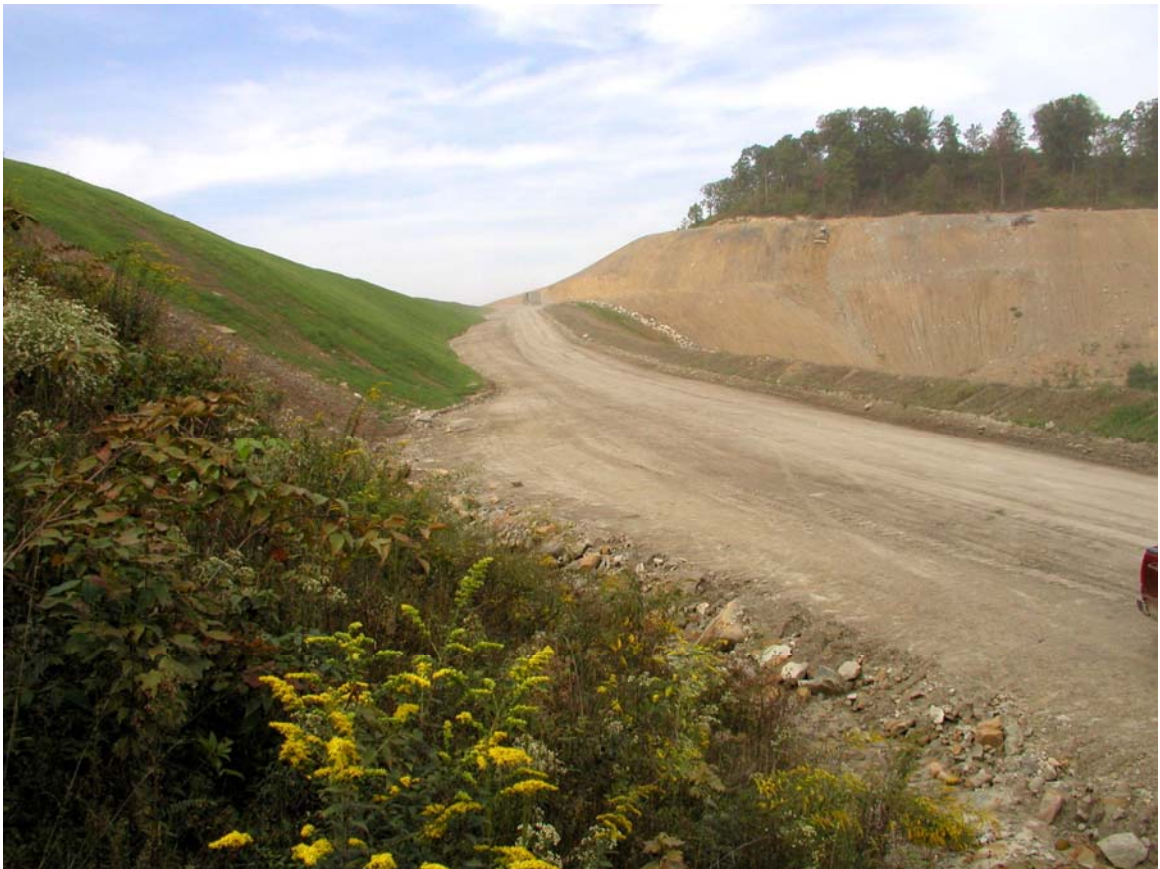
Figure 5. In the foreground is vegetation derived from a native seedbank, while the background is a conventionally hydroseeded bank at Pritchard Mine, WV, 2003.
