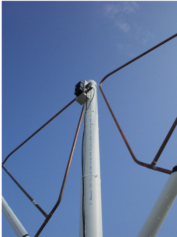
Figure 3.7: Picture of preamplifier installed at antenna terminals.
