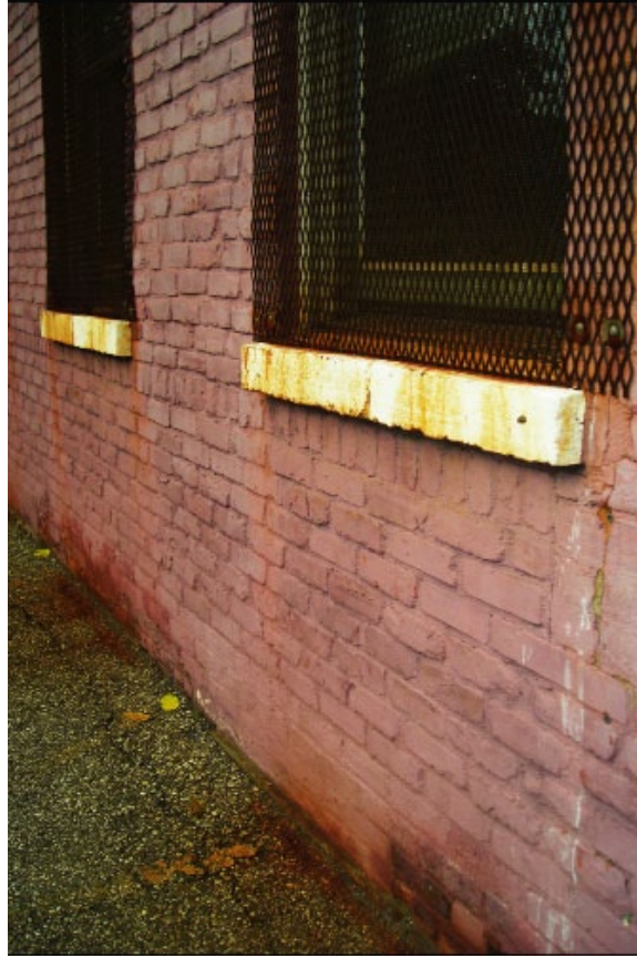
Picture of existing building on site
