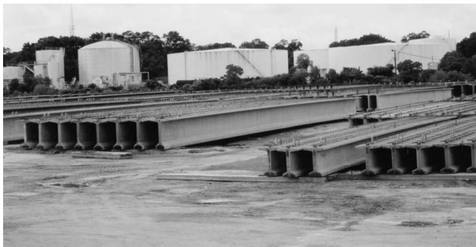
Figure 3.1: Beams Stored in the Casting Yard
