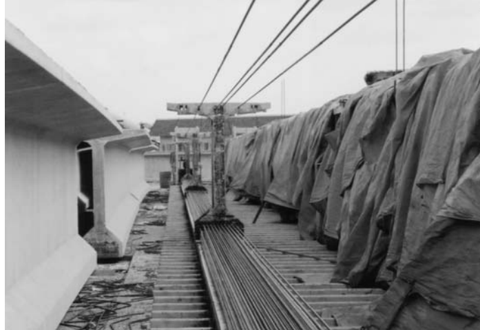
Figure 3.18: Beam with Strands in Casting Bed
