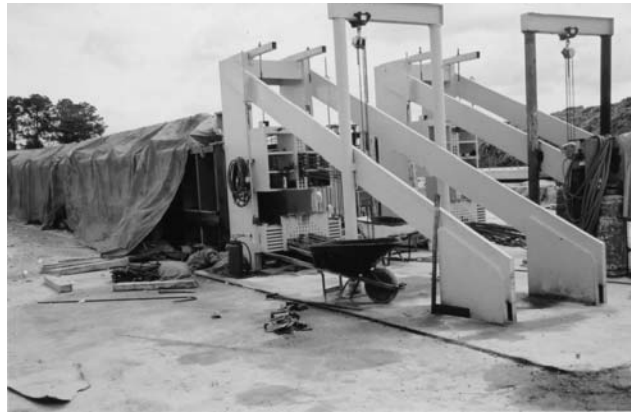
Figure 3.19: Beam Curing in Casting Bed
