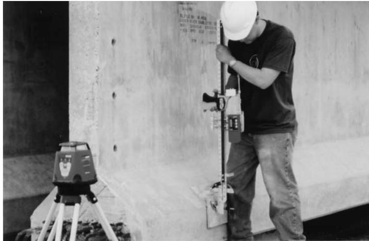
Figure 3.20: Taking Readings with Laser Level Surveying System
