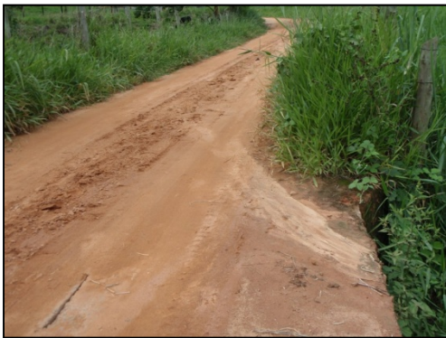
Figure 4.5. Example of direct delivery of sediment from a road segment evident by the flow patterns.
