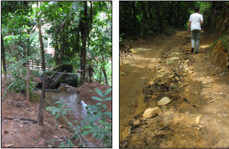
Figure 4.23. Photos of road segment 94 which received scores of 5 for both sediment production and sediment delivery using the field classification system.
