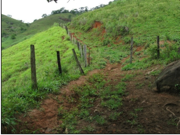
Figure 4.6. Road segment classified as ‘abandoned’ due to significant erosion and multiple gullies.
