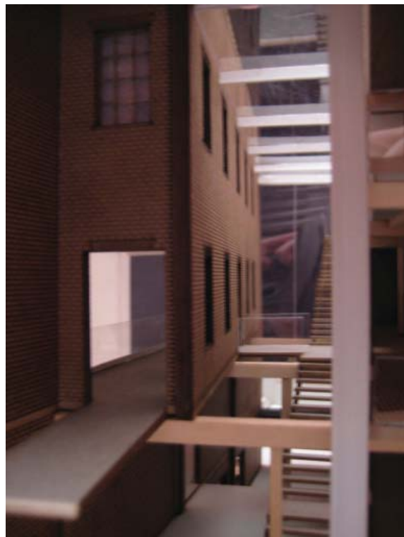
The original steel columns and concrete beams on the first level of the new atrium have been left completely intact as support for the angled masonry wall that creates the existing second and third level light well.
