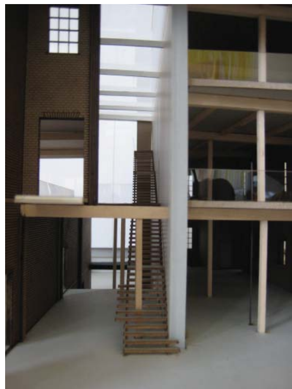
The original steel columns and concrete beams on the first level of the new atrium have been left completely intact as support for the angled masonry wall that creates the existing second and third level light well.
