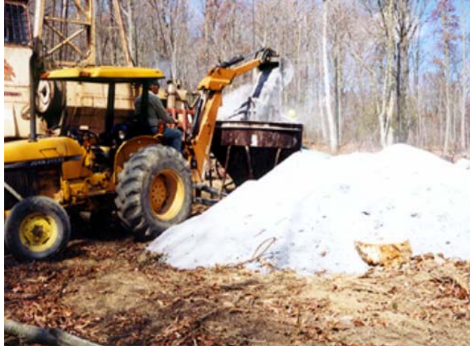
Figure 17: Tractor-mounted backhoe loading the bucket with lime.
