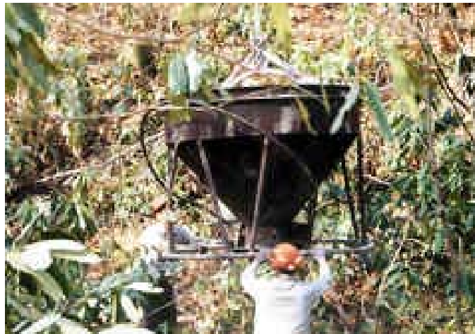
Figure 18: Two chokermen line up the bucket before opening the faucet in order to place the lime
