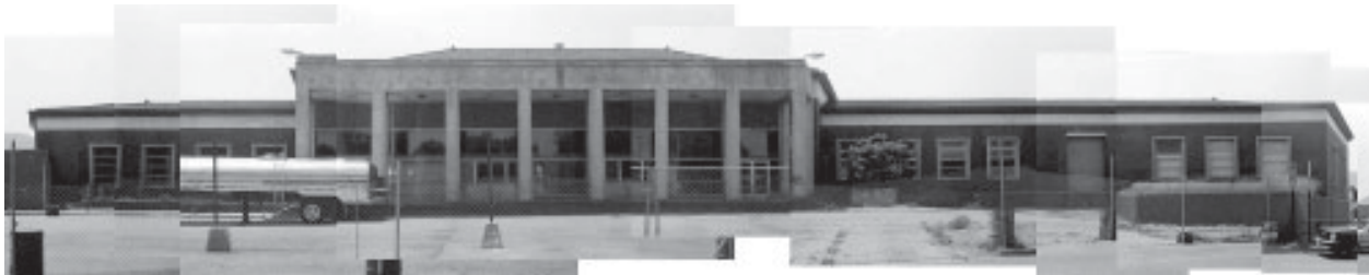
Norfolk and Western Passenger Train Station, Norfolk and Western Railroad, Built in 1905
