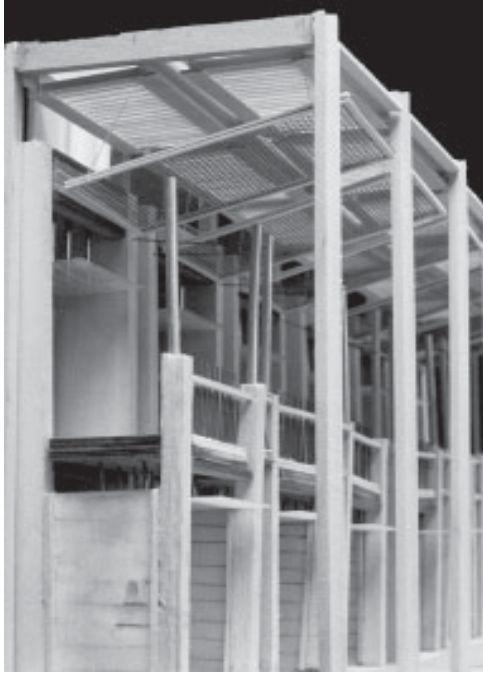
View down the atrium Drop ceilings aid to screen the upper and lower walkways from any direct sunlight.
