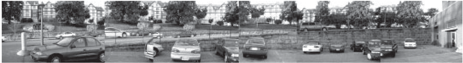
Existing retaining wall that encloses the north side of the courtyard
