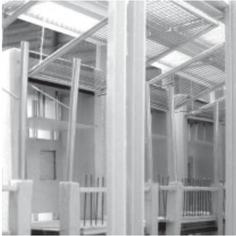
Screens aid to direct the air flow towards the return air duct. Ducts are located above each gallery unit on the top floor.
