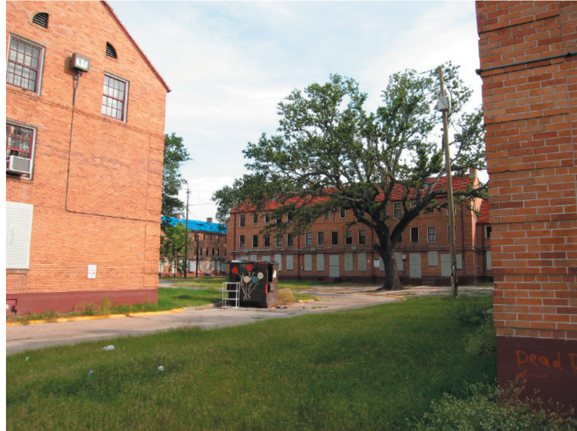
Site, Empty Courtyards July 2006
