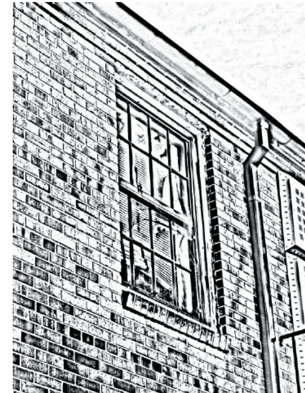
Existing Window Postedited Photograph, July 2006
