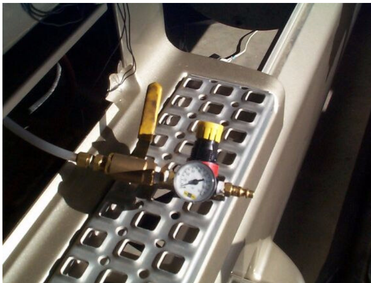
Figure 3-8. Inlet to Air Dryer
