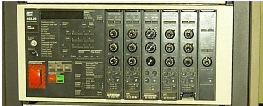
Figure 3-9. MTS 458.20 Hydraulic Controller
