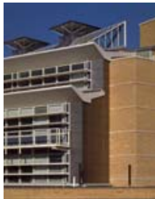
Figure 2.5 - Detail of wind towers at Ionica Building (“Ionica”)
