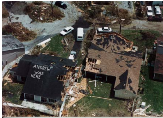
Figure 1.1 - Roof damage from hurricane Andrew (Rappaport, 2003, p. 3)
