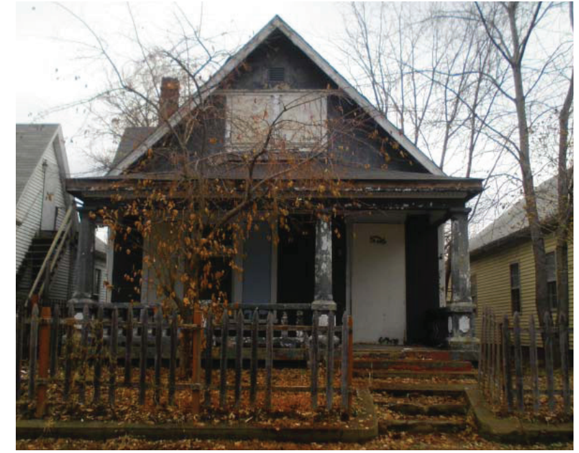
15 Abandoned Bates Hendricks Home
