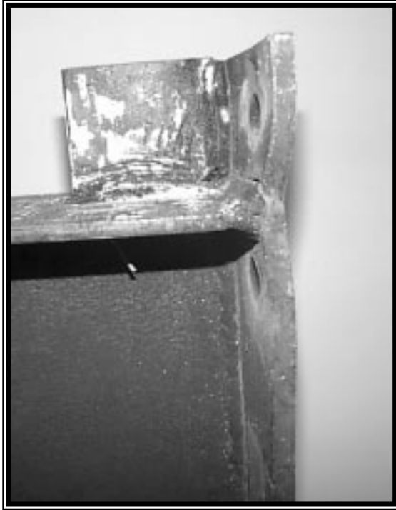
(a) Flange-to-End-Plate Fracture at the Weld
