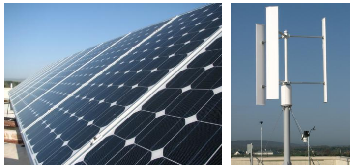
Figure 2.8: View of the CPES solar array and wind turbine mounted on the roof of Whittemore Hall, Virginia Tech, using Suntech 170W PV panels [source: www.suntech-power.com ], and Cleanfield wind turbine [source: www.cleanfieldenergy.com ]. Photos by CPES, 2008.
