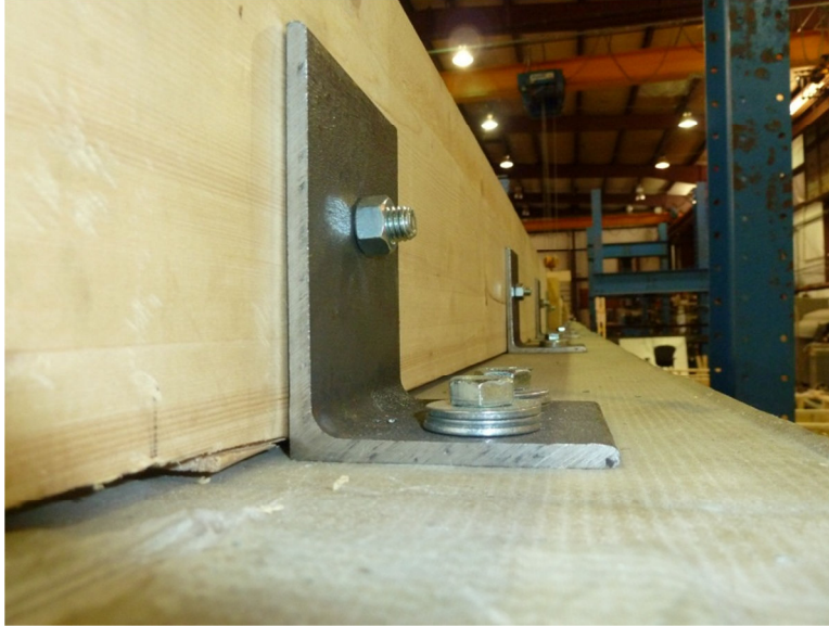
Figure 4-21 Deck Side Walls
