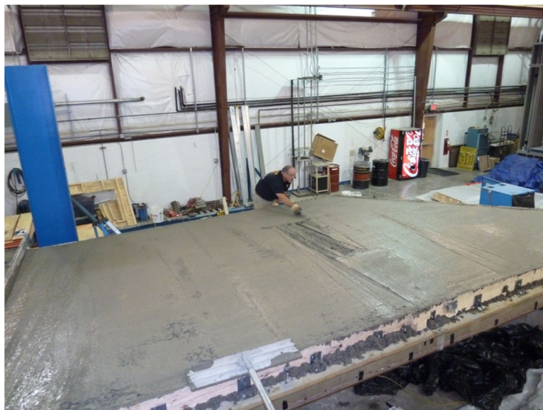
Figure 4-25 Finishing Done by Hand and Bullfloat
