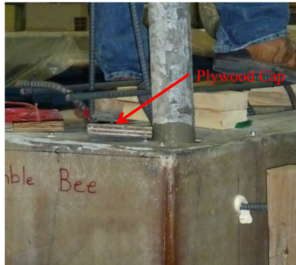
Figure 4-9 Plywood Cap at End of HCB
