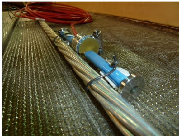
Figure 3-22 Installation of VWG on Bottom of Arch
