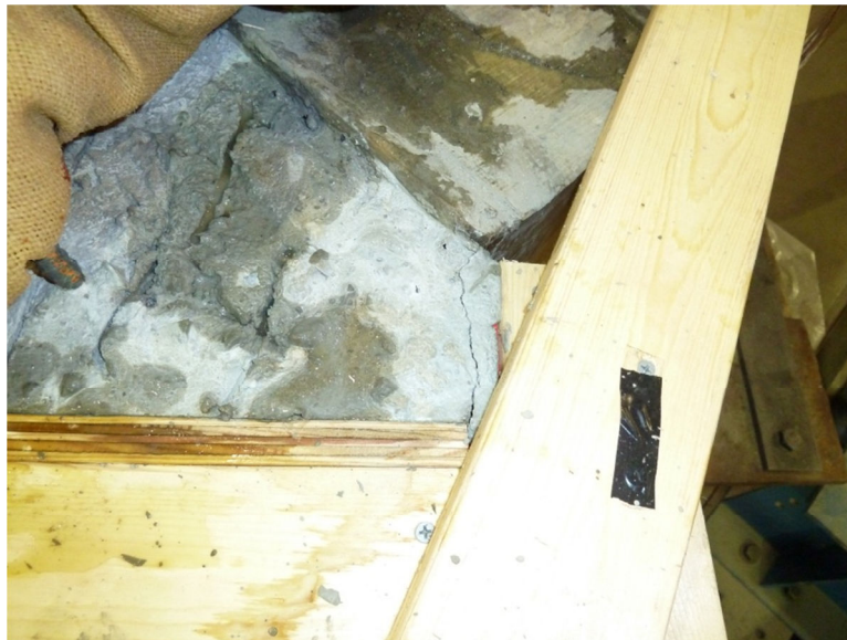
Figure 4-20 Roughened Diaphragm Surface
