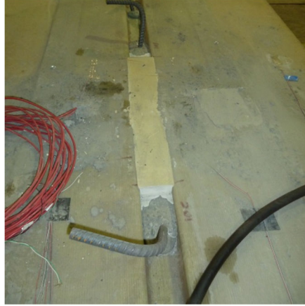
Figure 4-14 Plaster Placed in Channel of HCB
