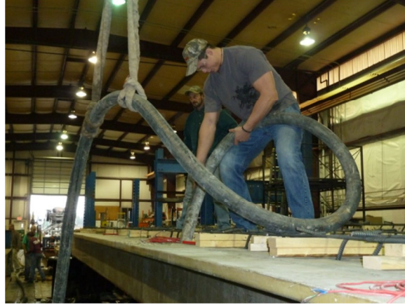
Figure 4-12 Concrete Pumped into Hole at Quarter Point
