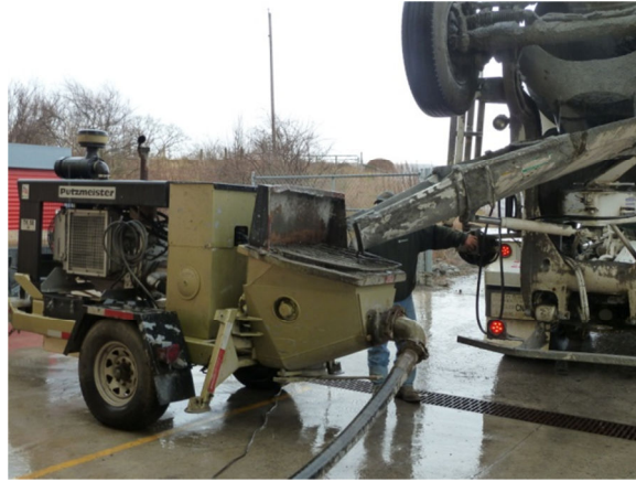
Figure 4-11 Concrete Pump Used for Arch Pour
