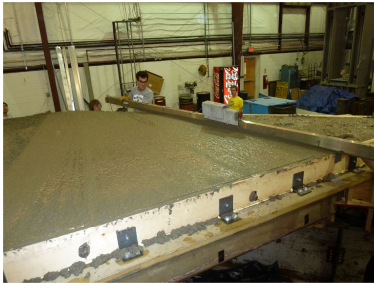
Figure 4-24 Screeding of Deck
