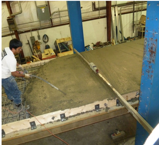
Figure 4-26 Edge of First Concrete Truckload
