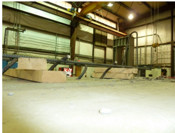
Figure 4-7 Reinforcement Tied to Shear Connectors
