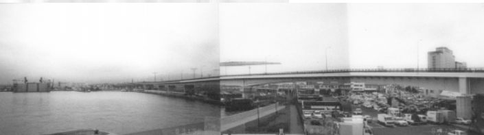
View toward the site across the elevated road
