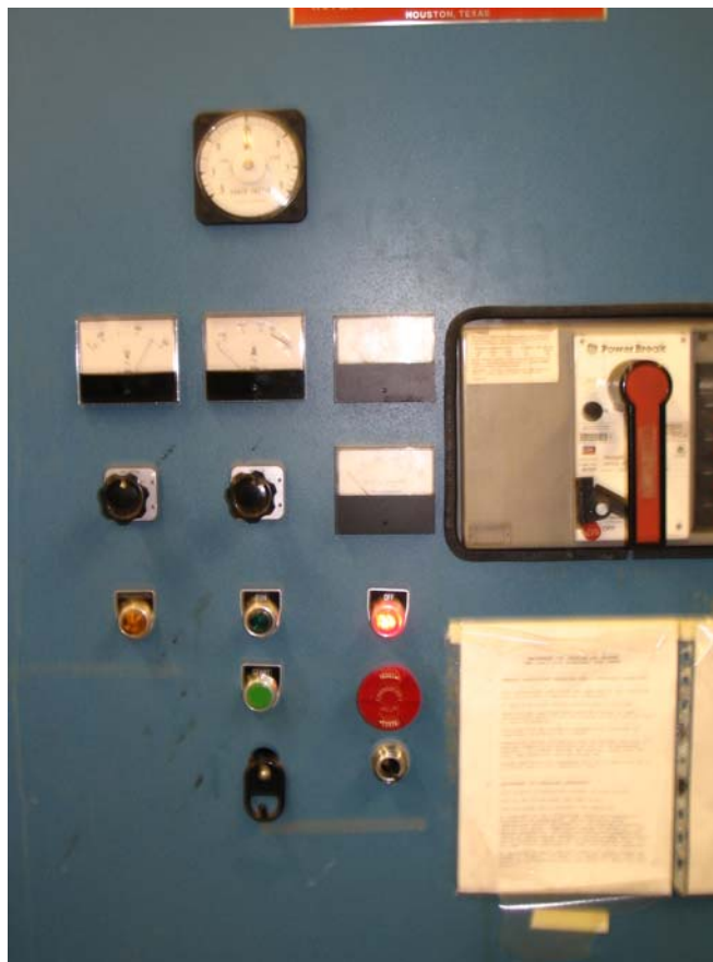
Figure D-2. Large blue air compressor control panel in the rear left corner of the compressor room.
