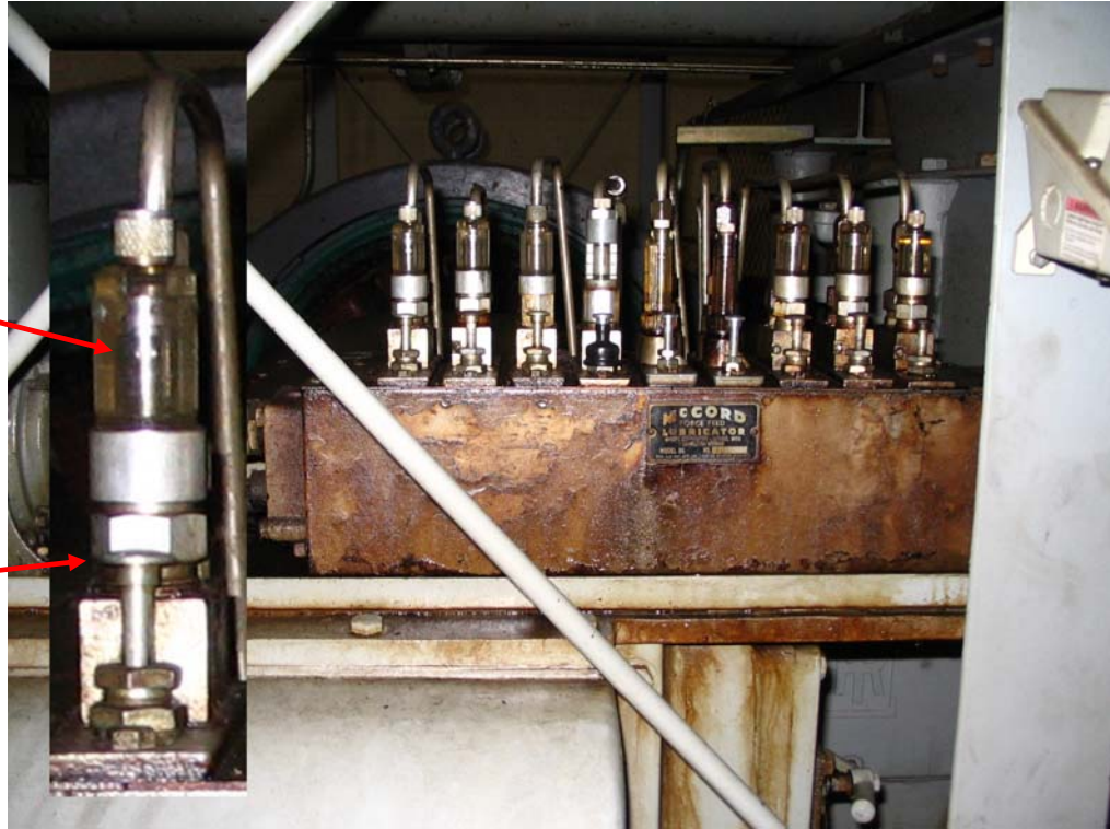
Figure D-3. Check compressor oiler for correct operation by observing an oil droplet in each of the nine oilers.
