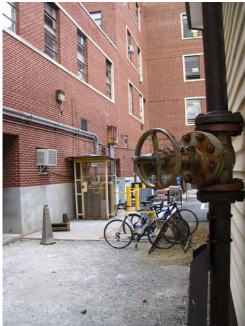
Figure D-11. Outdoor valve controlling air delivery to the ME Department side of Randolph Hall.
