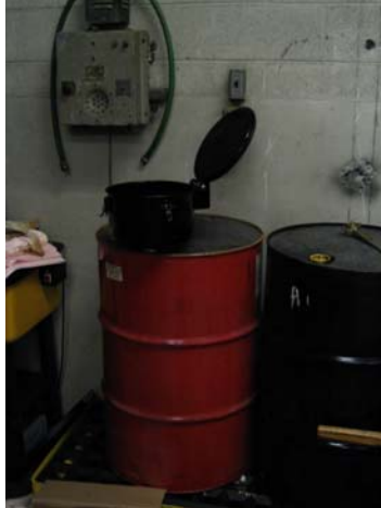
Figure D-10. Drum containing waste condensate oil/water mixture, located on rear wall of compressor room.
