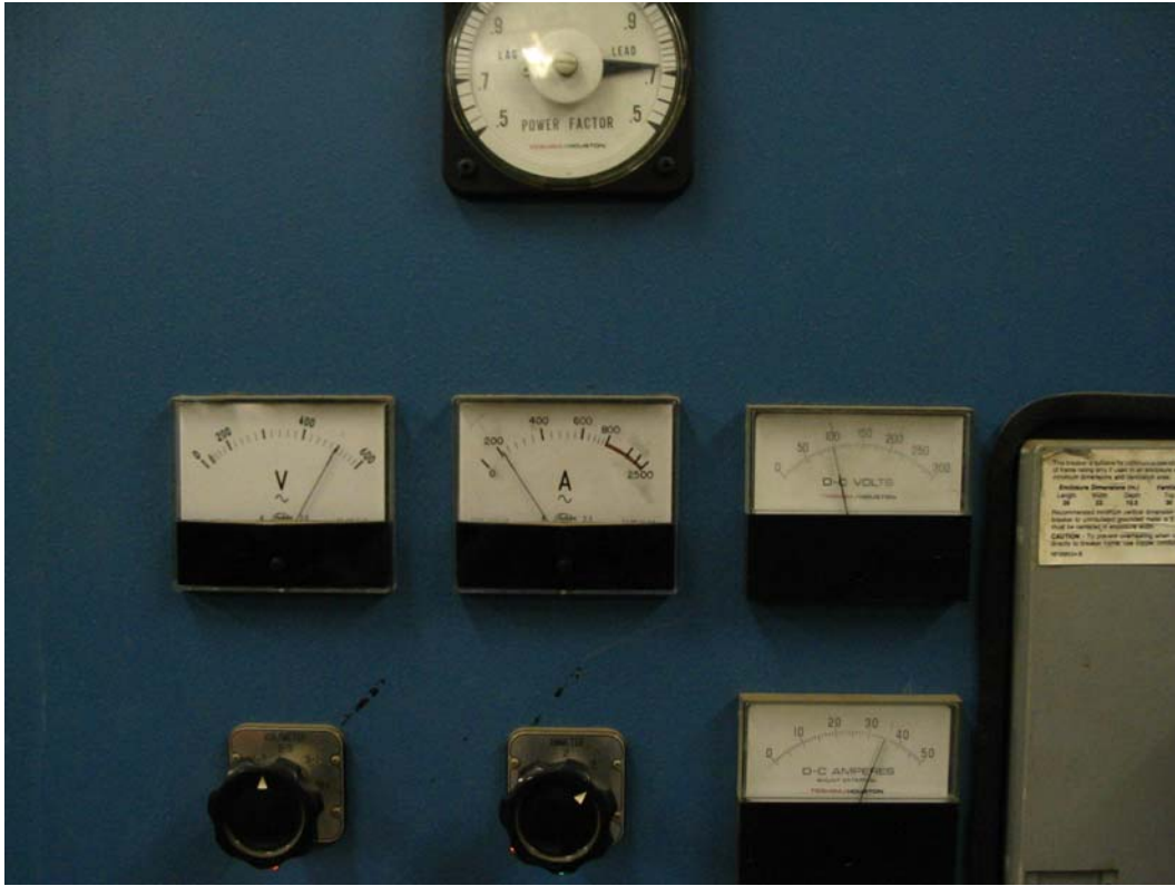
Figure D-6. After starting the compressor, check the gauges for proper indications, as discussed.
