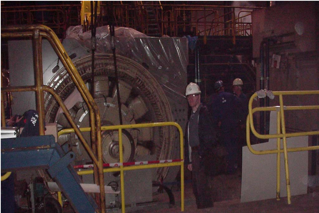
Figure 1-2; The author in a former life, working on an 11 MW, 6.6 kV AC induction motor. The cooling and lubrication systems are not installed, but the cooling water lines and heat exchanger can be seen atop the unit to the right. Total volume is about 60 m 3 , the rotor alone masses about 23 MT and the stator another 36 MT.
