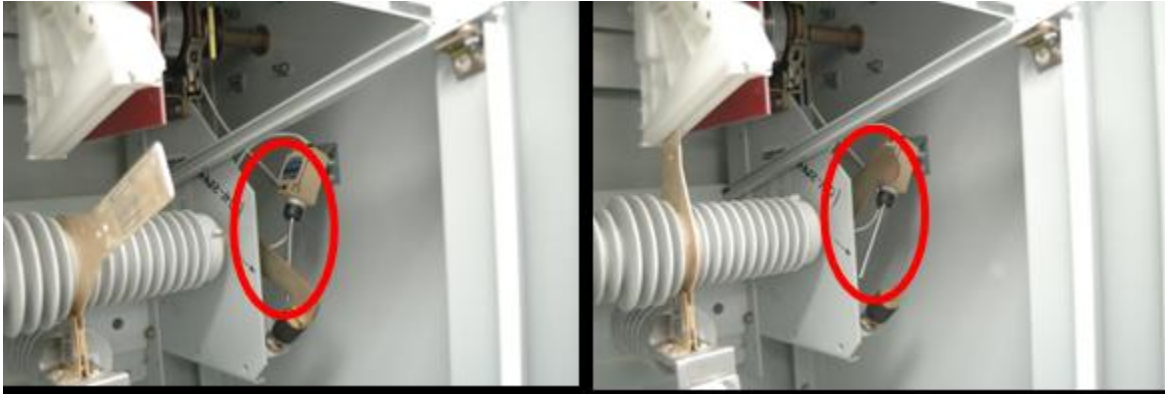
Figure 3-3; High voltage switch status sensor "open" and "closed."
