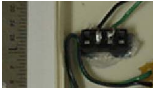
Figure 3.5.4.2. Battery connection terminal.
