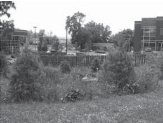
Storm-water Retaining Pond
