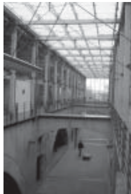
Lyon School, Interior
