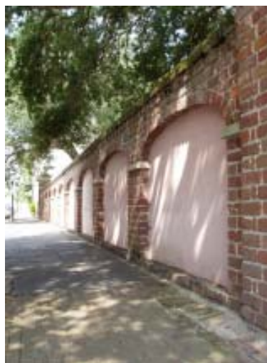
Brick walls surrounding site
