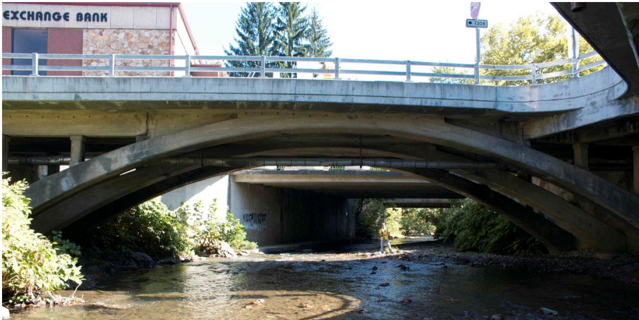
Figure 1-7. Depot Street Bridge from Upstream
