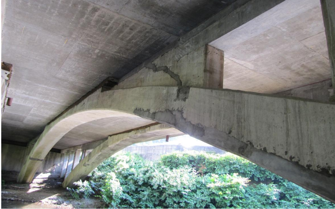
Figure 1-9. Patched Concrete Arch Cracks
