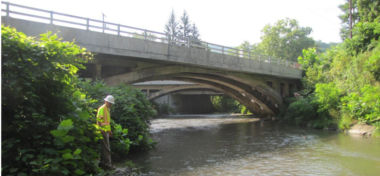
Figure 1-4. Main Street Bridge from Upstream
