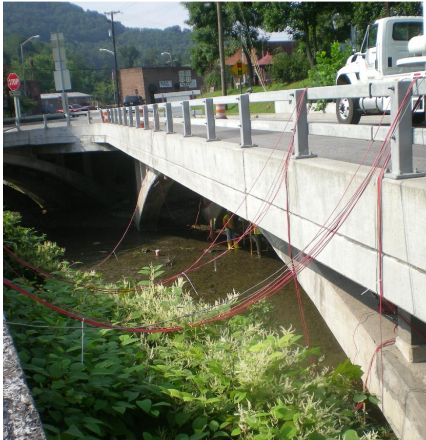
Figure 3-10. Bridge Instrument Wiring
