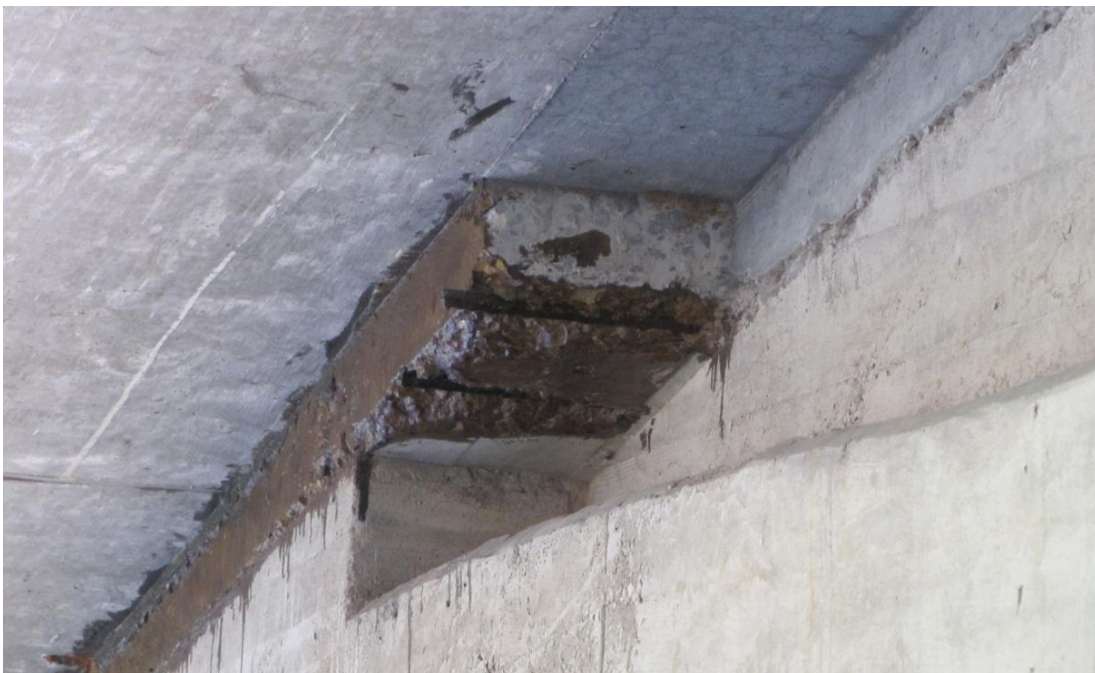
Figure 1-10. Steel Reinforcement Corrosion
