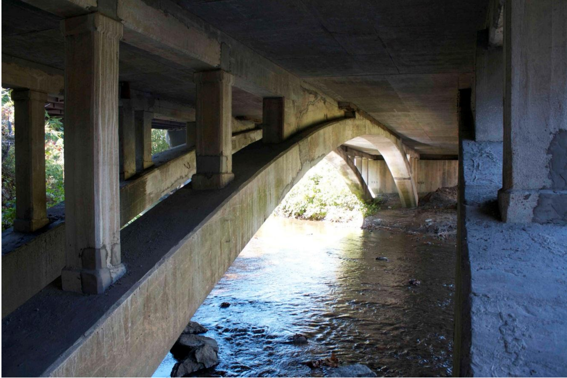
Figure 1-5. Bridge Superstructure
