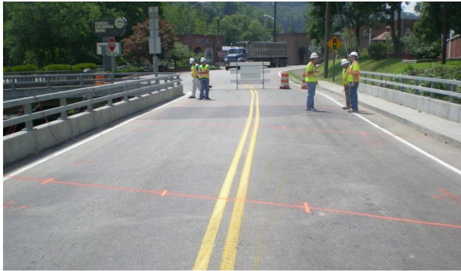
Figure 3-19. Truck Reference Lines on Bridge Deck
