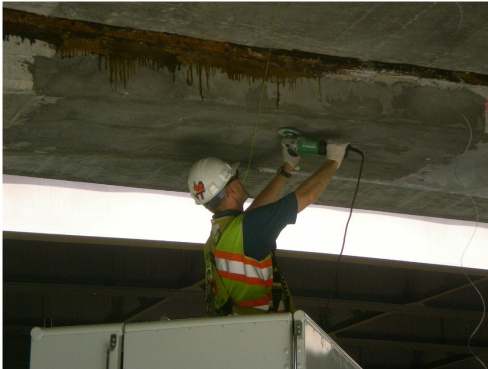
Figure 3-2. Smoothing Concrete Arch Surface with Grinder
