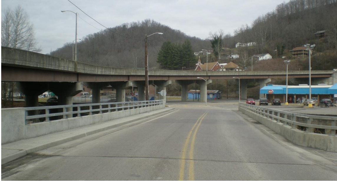
Figure 1-6. Traffic Lanes of Main Street Bridge
