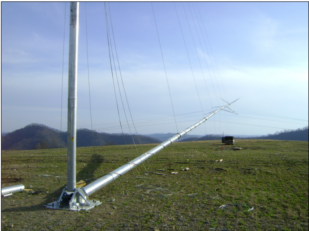
Figure 3.10 – White Flame #10 Tower Installation I
