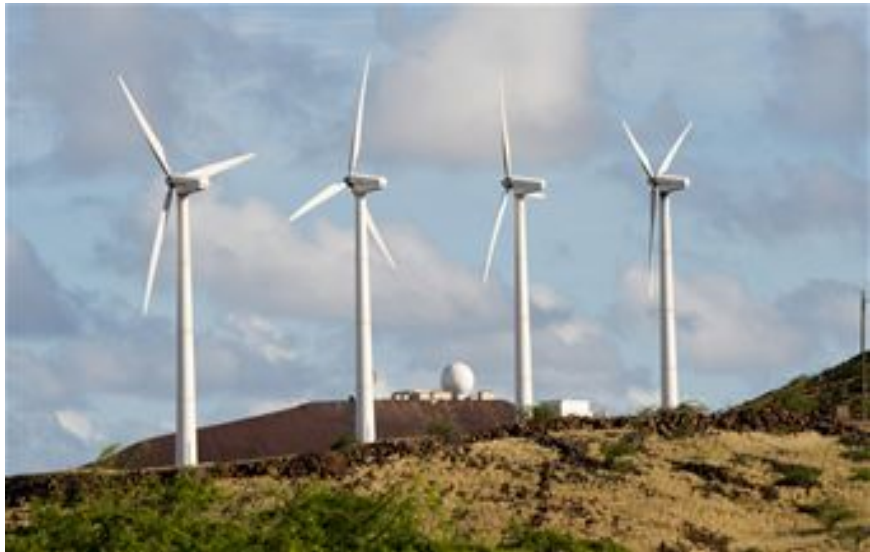
Figure 9: Four 225 kW Turbines at Ascension Island (INEEL 2004) ( http://www.windpoweringamerica.gov/winddiesel/pdfs/2004_wind_diesel/operational/dod.pdf ) (public domain)
