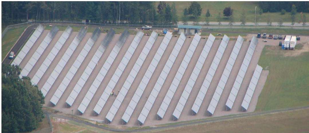
Figure 11: Burlington ANG Ground Mounted Array (Burlington ANG 2011) ( http://www.engineersconstruction.com/projects/vtang-solar/ ) (public domain)
