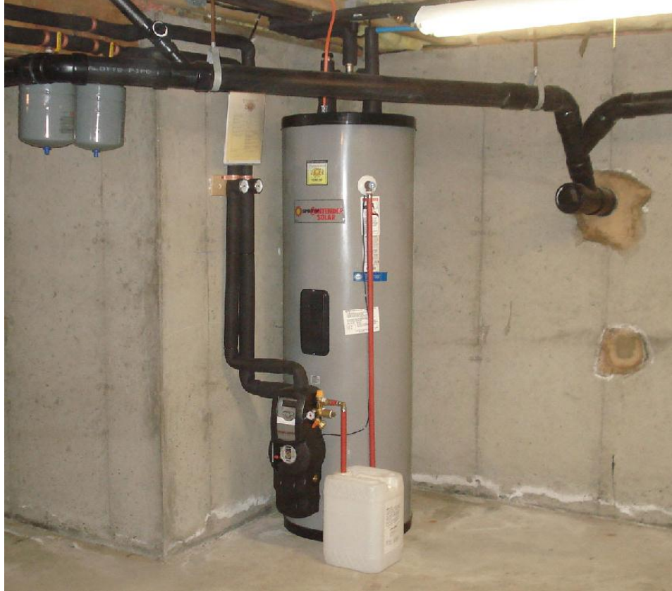
Figure 4.8 Photo of a solar water heater with internal heat exchanger and solar control station attached to the storage tank (Courtesy: www.renewedbytheson.com )
