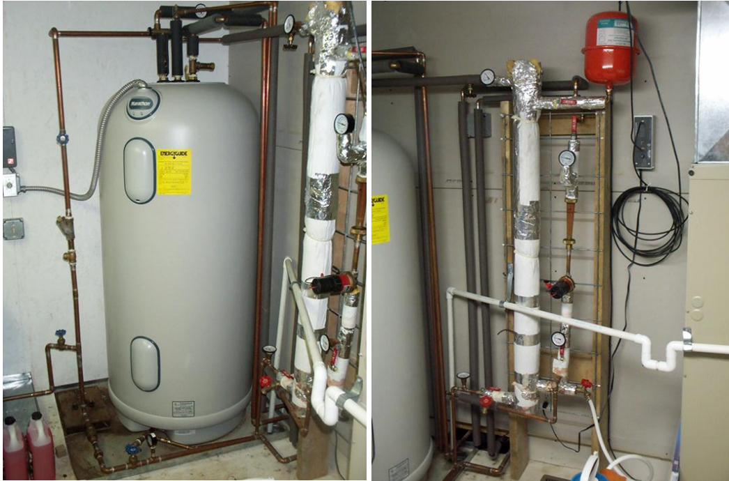
Figure 4.7 Photo of a solar water heater tank with external heat exchanger in white on the right side of the tank (Courtesy: www.renewedbytheson.com )
