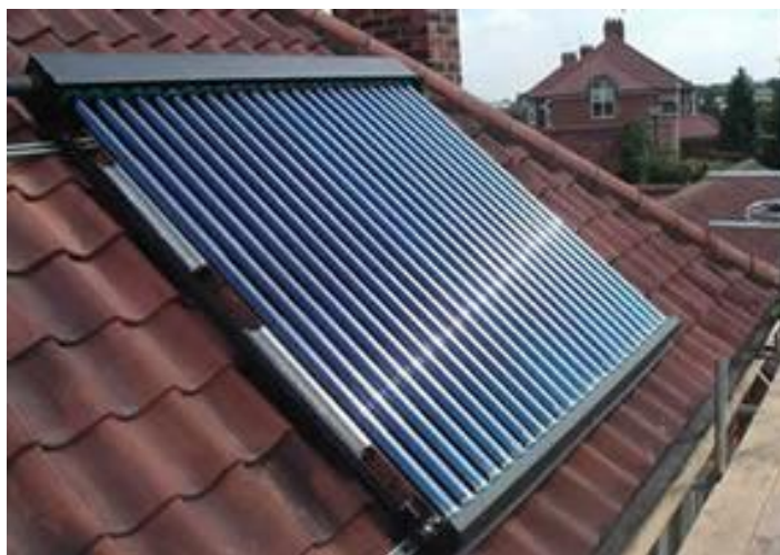
Figure 4.3 Top frontal view of a commercially available evacuated glass tube collector
