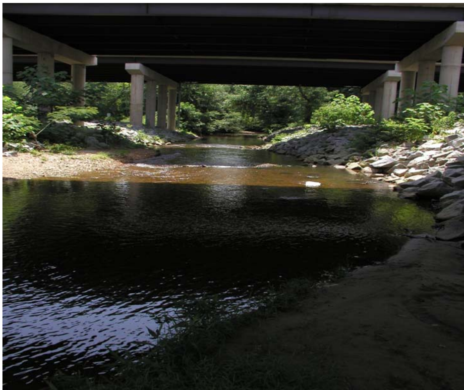
Site Q8: The single lane bridge is adjacent to a larger four lane bridge.
