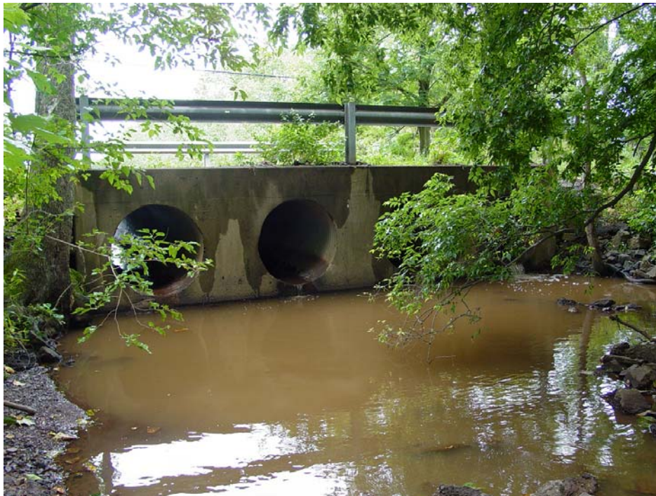
Site Q10: The two lane bridge featured generally low traffic.
