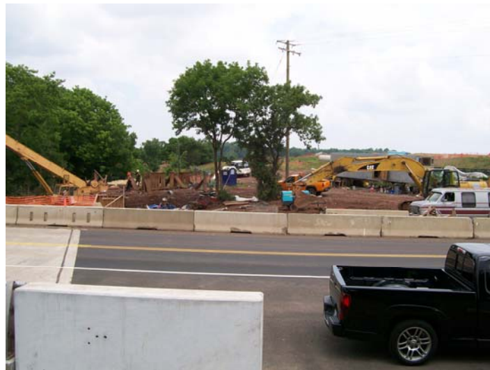
Site Q16: An example of the ongoing bridge construction.
