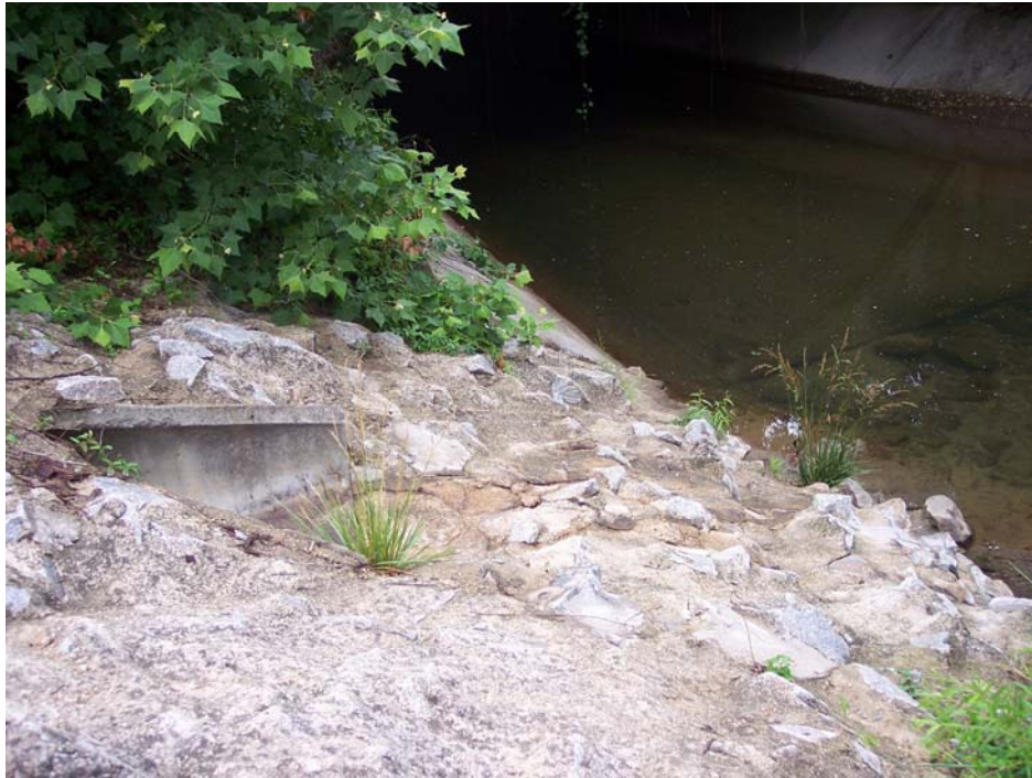
Site Q2: The storm drain leads directly to the creek.
