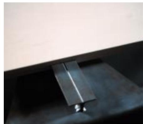
Table 3:1, topside, double angle/slot 'embracing' connection. Welded 'mounting' connection and lamination are also pictured. (detail photo).
