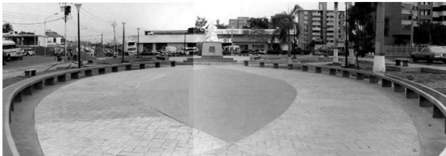
Figure 5 Plaza de la Madre deforested during renovation
