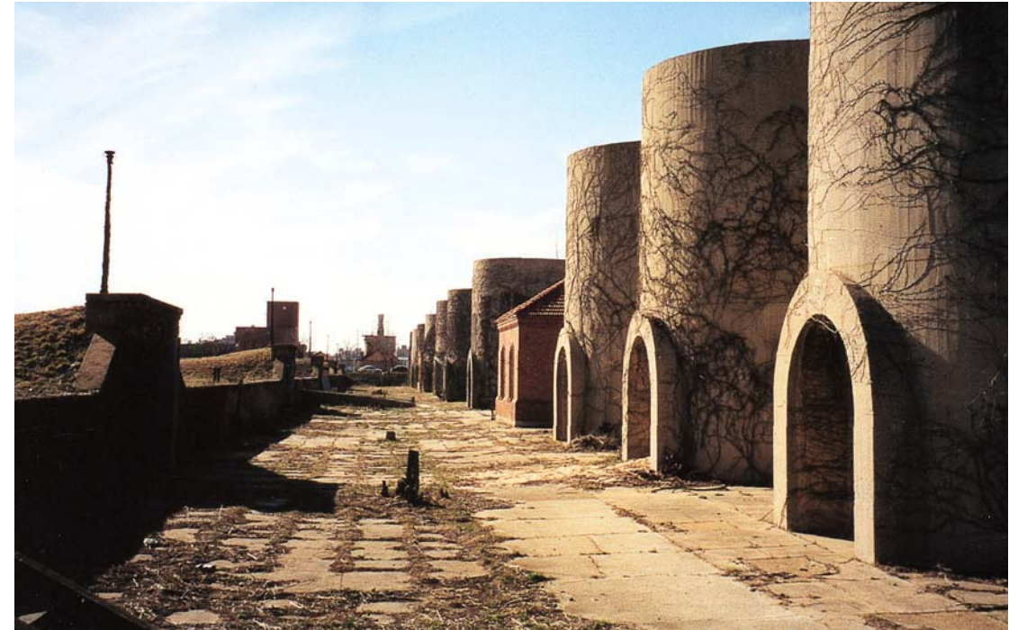
4.2 Service court with sand bin towers
