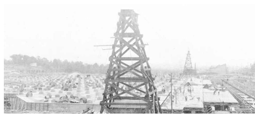
2.8 Site under construction
