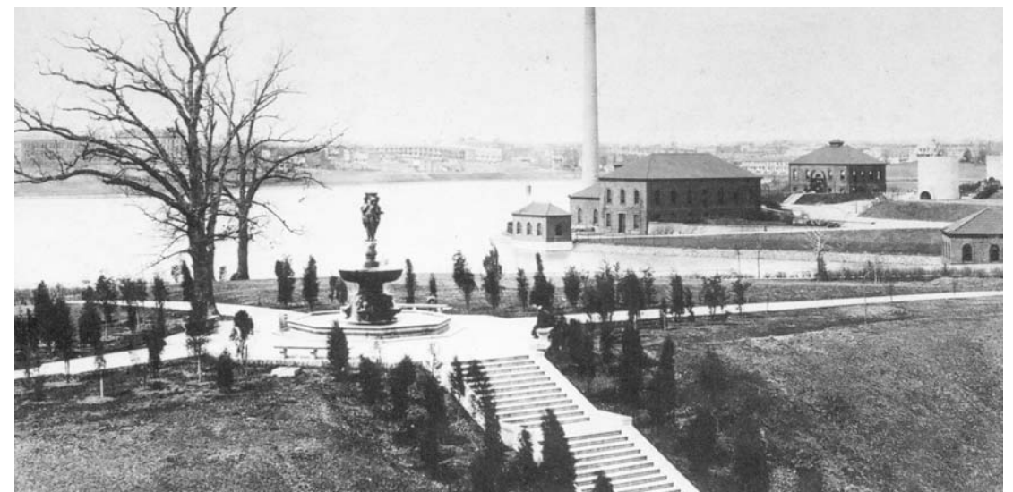
2.9 McMillan Fountain, Reservoir, and pumping station
