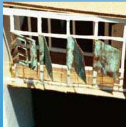
Process Model: Brise Soleil and french doors at residence wing
