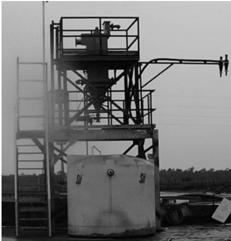
FIGURE 33: PILOT SCALE TESTING FACILITIES
