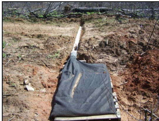
Figure 3. Dirtbags® installed on bladed skid trail.
