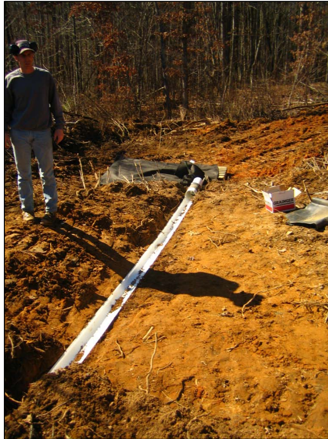
Figure 4. Gutter system installed at treatment base.
