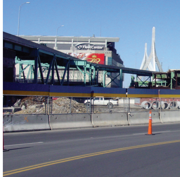
*2 construction of the Big Dig
