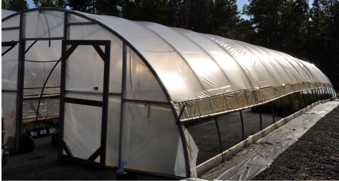
Figure 1.2 Quonset Style Cold-frame (Credit: William K. Harris)
