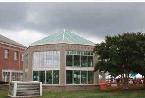
7: New City Hall Entrance
