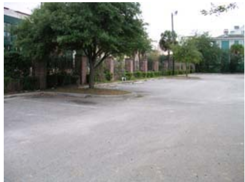
Figure 4.6. Existing parking lot in Charleston, SC showing current parking lot ordinance requirements.
