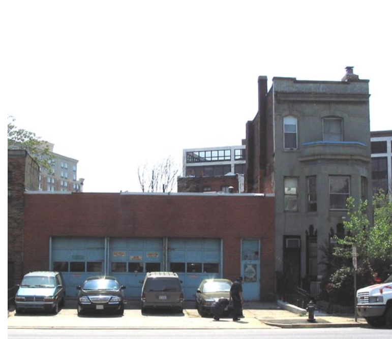
Auto body shop and a row house still used a single family residence along New York Ave. By Author
