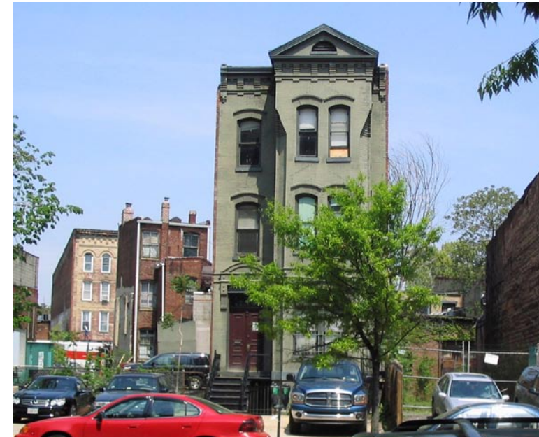
Row house or converted apartment building along K Street. By Author
