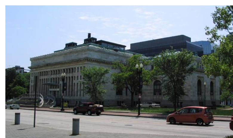
5. Old Carnegie Library, Formerly the Central Library of DC, Currently the National Music Center, North facade
