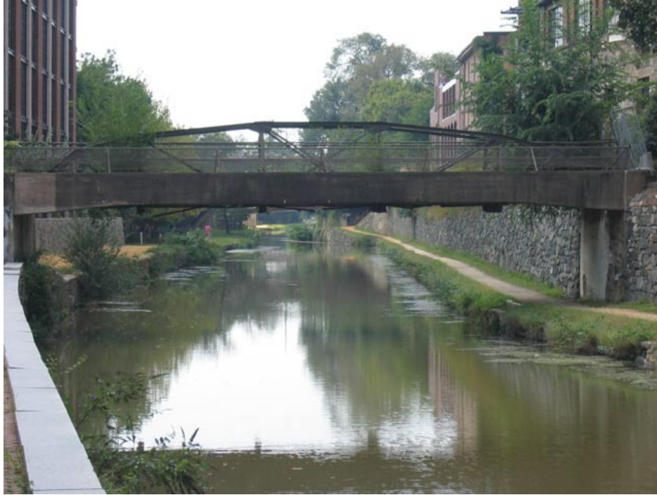
The site, C&O Canal Georgetown Looking North photo by Patrick Cooke
