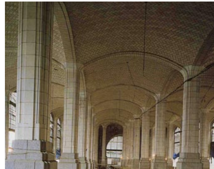
Fig. 7 Guastavino's tile vaults beneath the Queensboro Bridge, New York.
