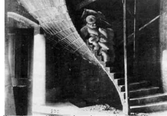
Fig. 1 Structural Test performed on spiral stairway First Church of Christ Scientists New York, 1900
