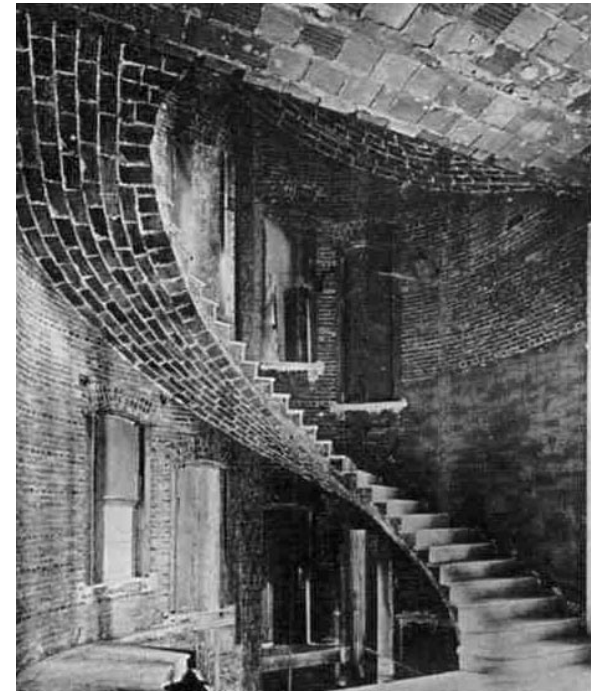
Fig. 2 Elliptical stair, First National Bank of Paterson New Jersey
