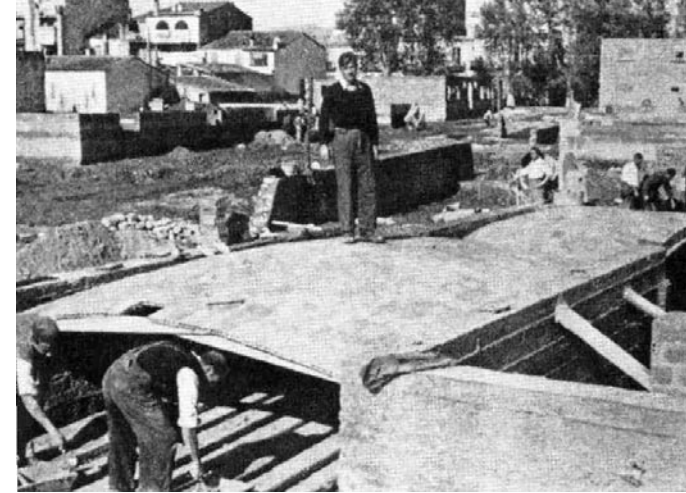
Fig. 6 Cohesive construction used to build a shallow vault with a single curved board as formwork
