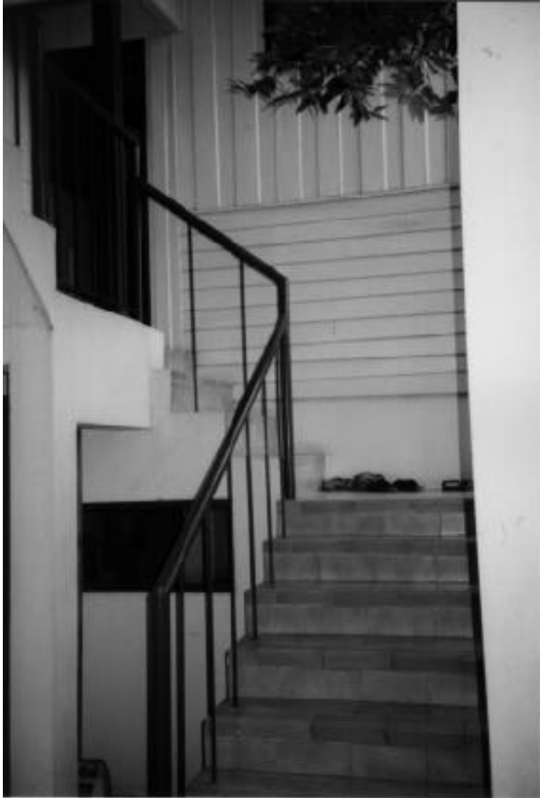
Figure 20. Built new stairs and stair landings
