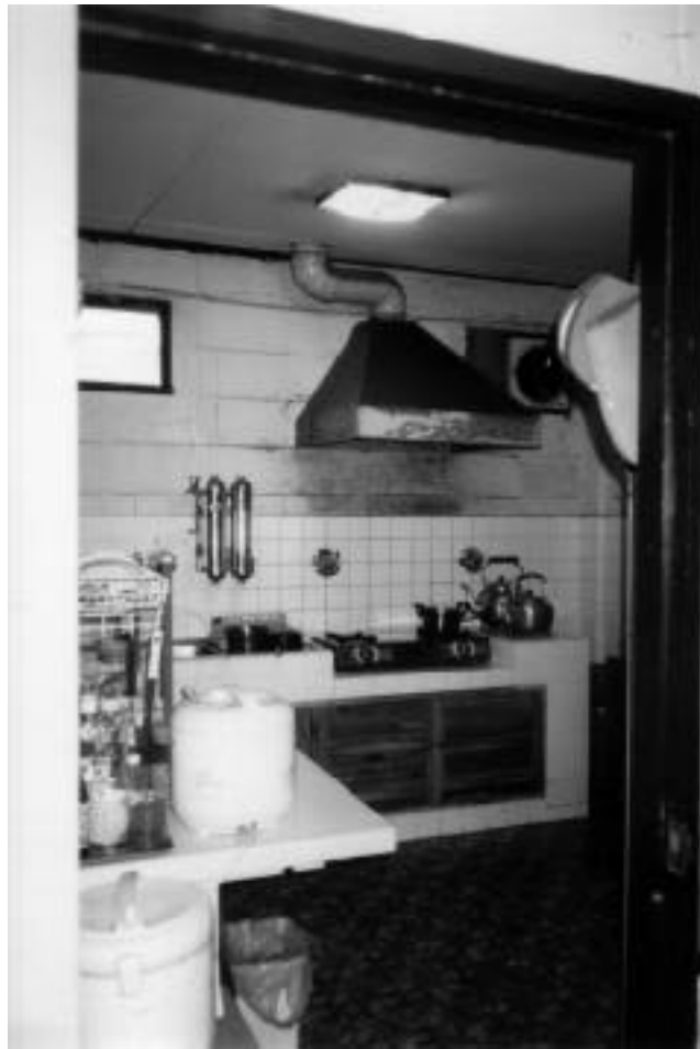
Figure 21. Installed a hood and an exhaust fan in the kitchen
