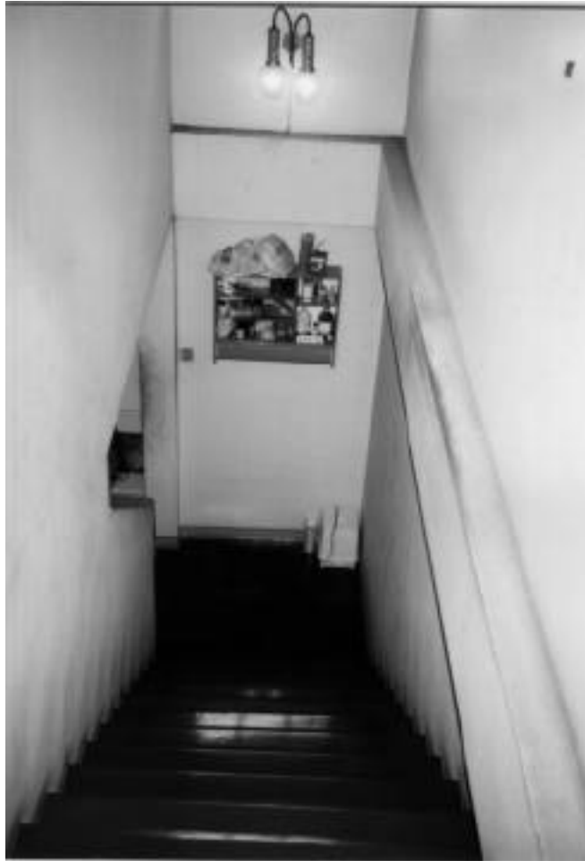
Figure 18. Steep stairs without railings
