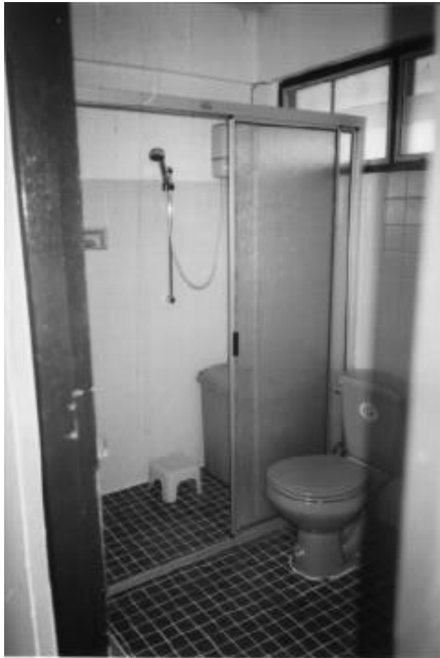
Figure 19. Replaced a toilet from an Eastern style to a Western style, added a shower seat, a shower door, a water container, and changed floor tiles in the bathroom
