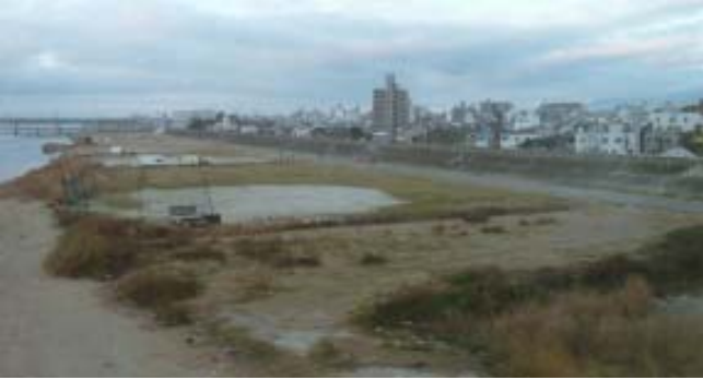
Playing fields and pathways contained within floodplain area of raised bermed river banks
