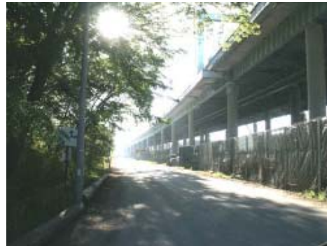
Shaded areas under bridge and forest canopy
