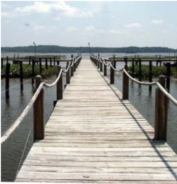
Example walkway to be used in tidal marsh areas
