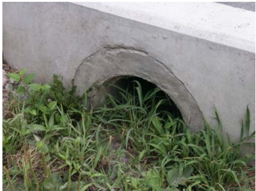
Water's influence on Jones Point north part of retaining wall (above) and under road (below)
