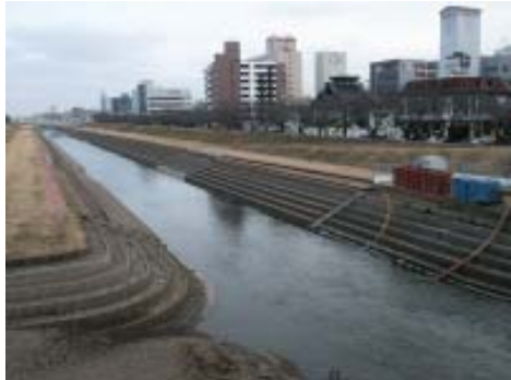
Engineered river bank edges typical through urban areas
