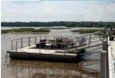
Picture of similar dock structure
