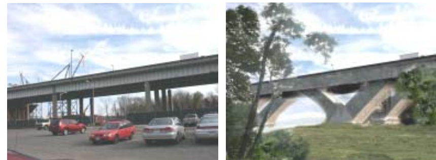
Comparison of present bridge (left) to a composite picture of perspective view of New Potomac River Bridge (right) from Jones Point
