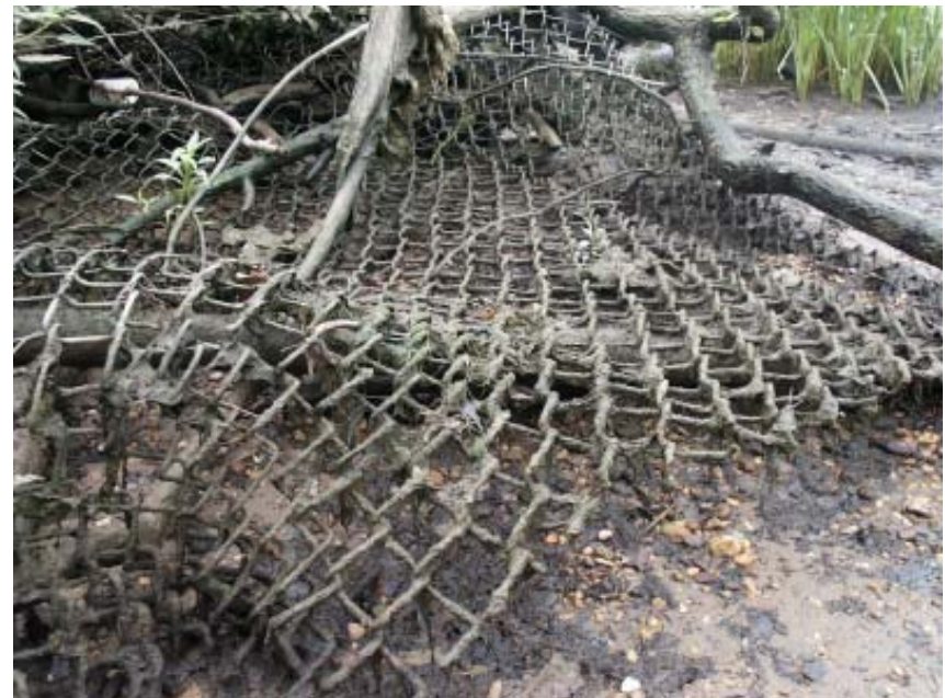
Views of the water-land transitional area around Jones Point park
