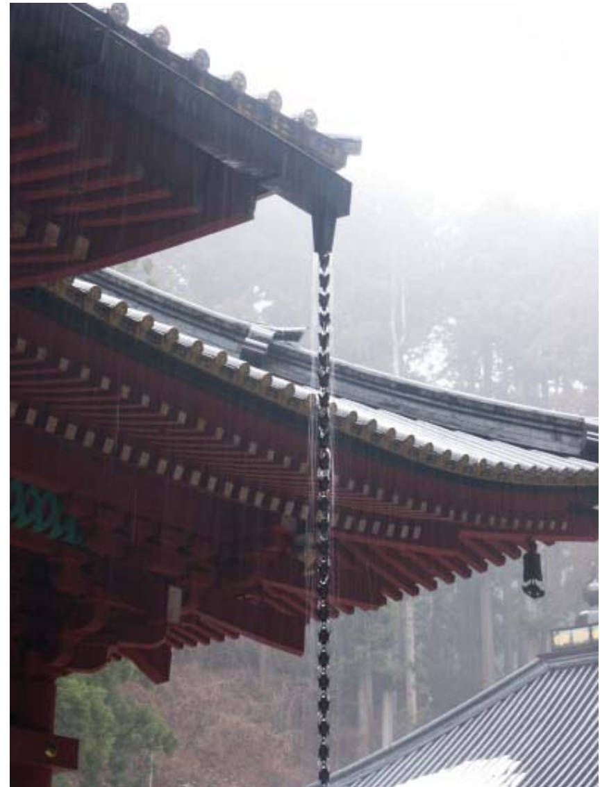
Downspout chain in Nikko, Japan (February 2003)
