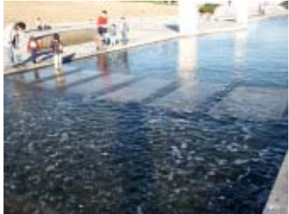
Submersible water crossing in circular amphitheater area
