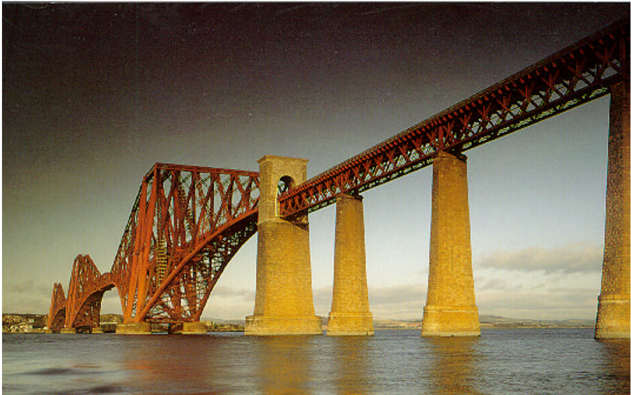
Figure 2-24: The Forth Rail Bridge, Great Britain (taken from Brown 1993, p72)
