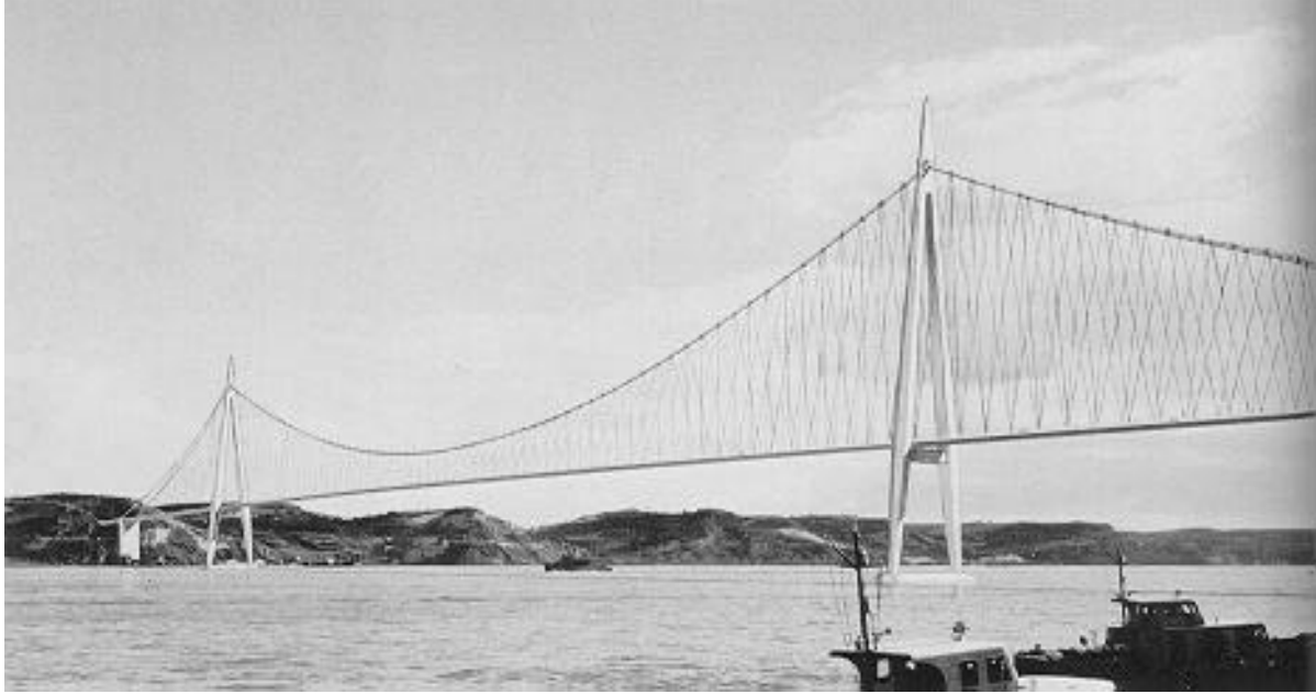
Figure 2-34: Monocable Suspension Bridge (taken from Leonhardt 1984, p292)
