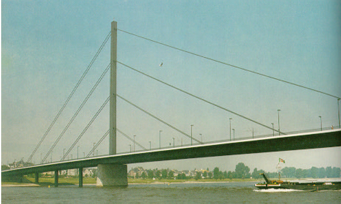
Figure 2-30: The Oberkassel Rhine Bridge, Düsseldorf, Germany (taken from Leonhardt 1984, p260)
