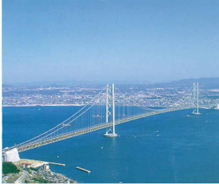
Figure 2-33: The Akashi Kaikyo Bridge, Japan (taken from Honshu-Shikoku Bridge Authority 1998, p1)
