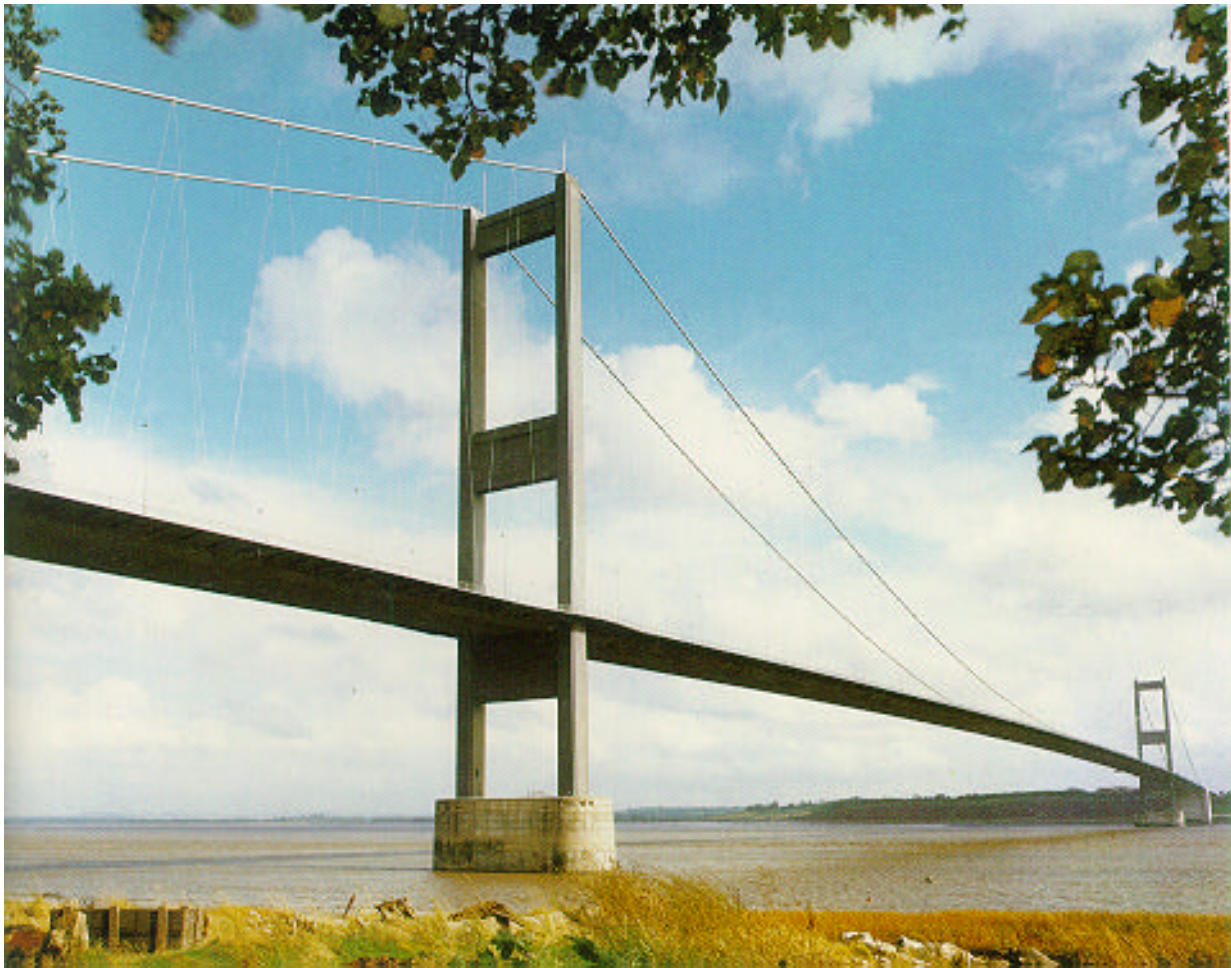
Figure 2-27: The Severn Bridge, Great Britain (taken from Leonhardt 1984, p293)
