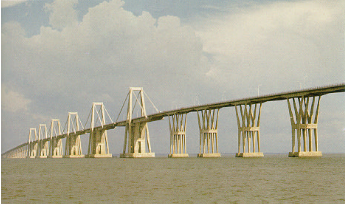
Figure 2-31: The Lake Maracaibo Bridge, Venezuela (taken from Leonhardt 1984, p271)
