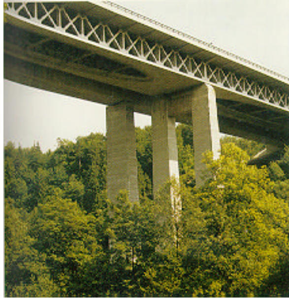
Figure 2-37: Concrete Trusswork in Mangfall Bridge, Austria (taken from Leonhardt 1984, p203)
