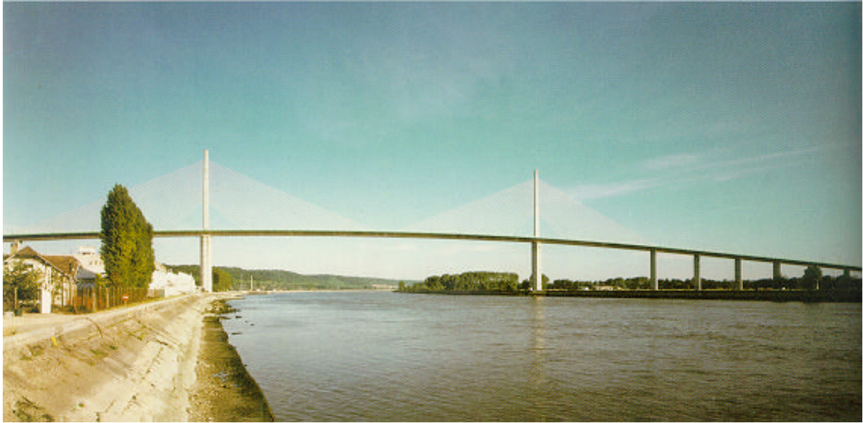
Figure 2-32: The Pont de Brotonne, France (taken from Leonhardt 1984, p270)
