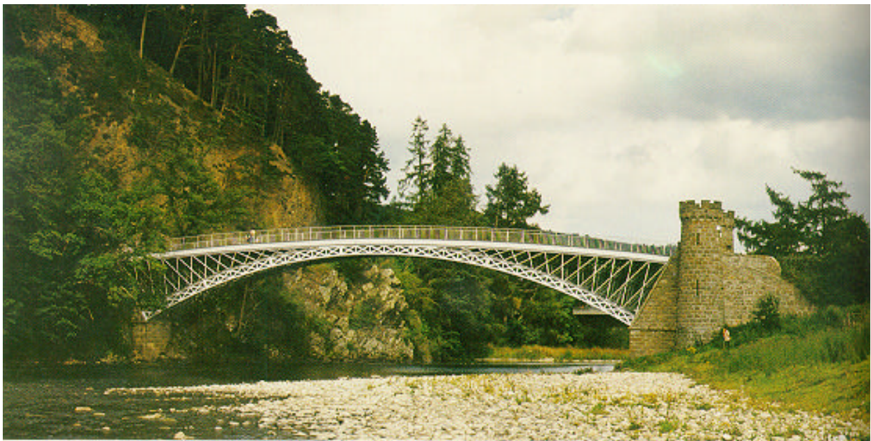
Figure 2-16: The Craigellachie Bridge, Great Britain (taken from Leonhardt 1984, p222)
