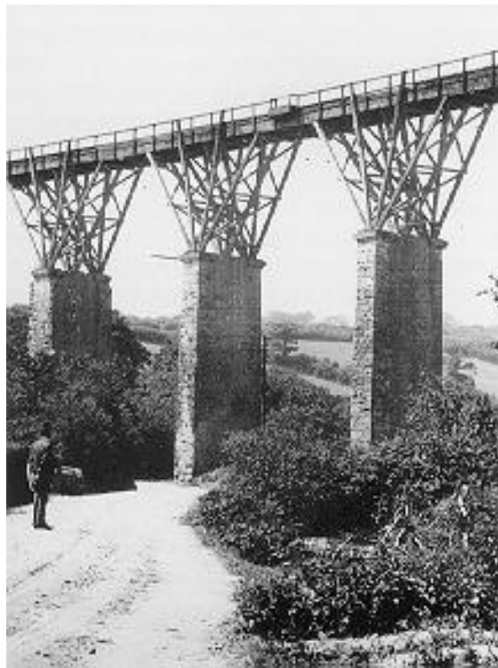
Figure 2-21: Timber Railway Viaduct (taken from Brown 1993, p66)
