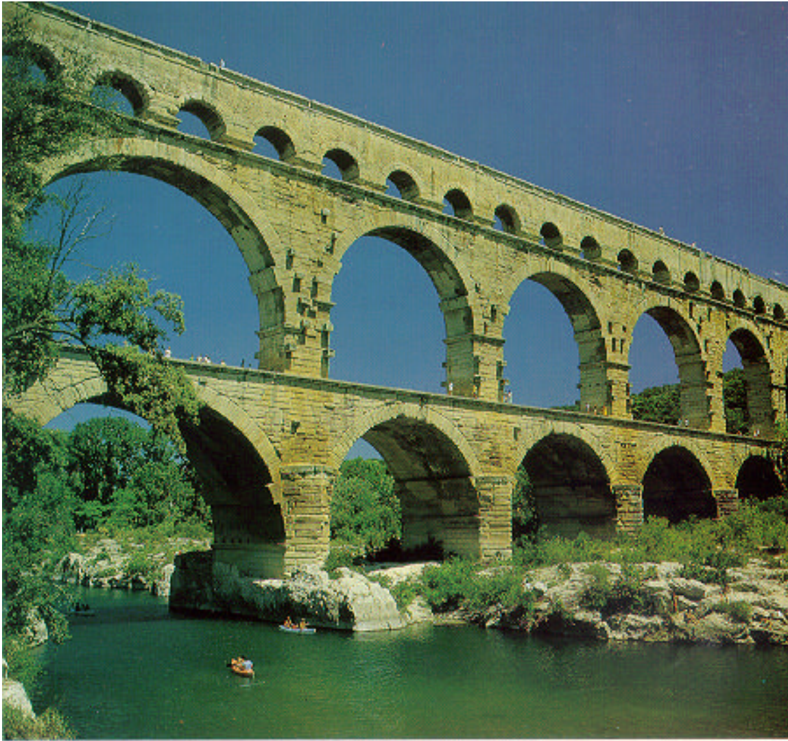
Figure 2-2: The Pont du Gard, Nîmes, France (taken from Brown 1993, p18)
