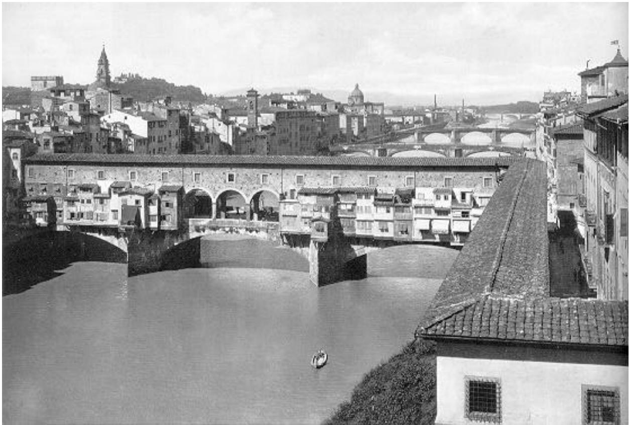
Figure 2-7: The Ponte Vecchio, Florence, Italy (taken from Leonhardt 1984, p75)
