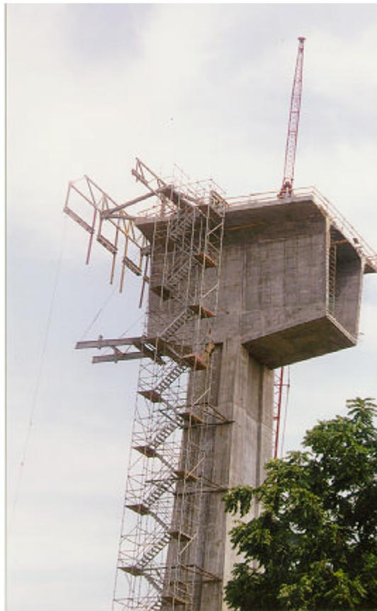
**Figure 3-3: Pier and Pier Table Design of the Wilson Creek Bridge**
