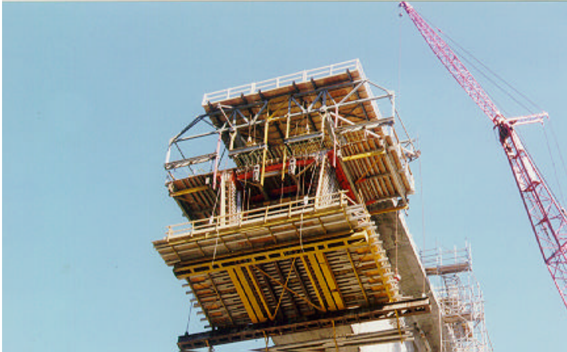
Figure 5-24: Form Traveler Detail
