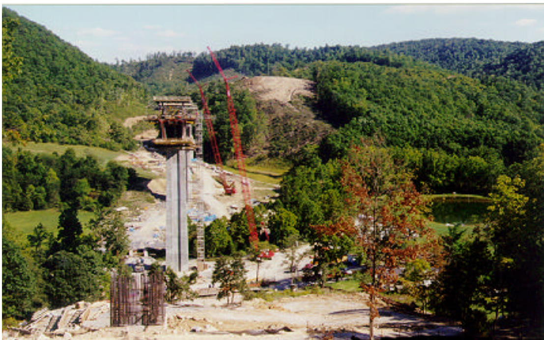
Figure 5-14: Site Overview from Abutment A
