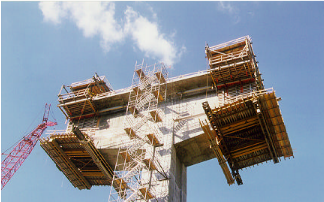
Figure 5-23: Beginning of Cantilevering Operations about Pier 2
