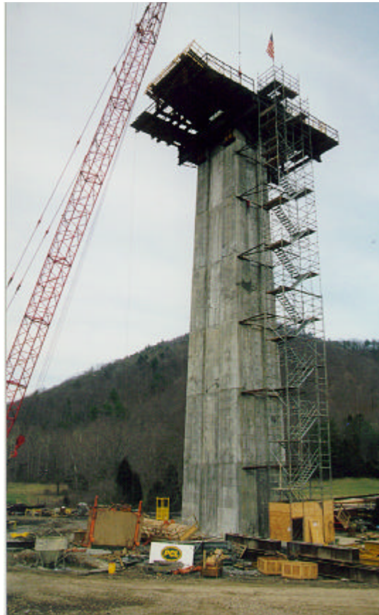
Figure 5-6: Pier 2 Prior to Construction of Pier Table
