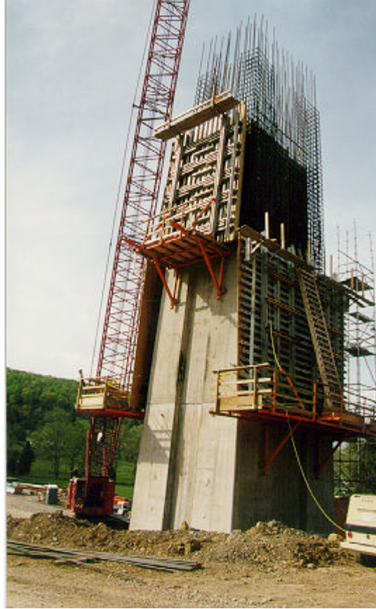
Figure 5-16: Pier 3 During Construction with Climbing Formwork
