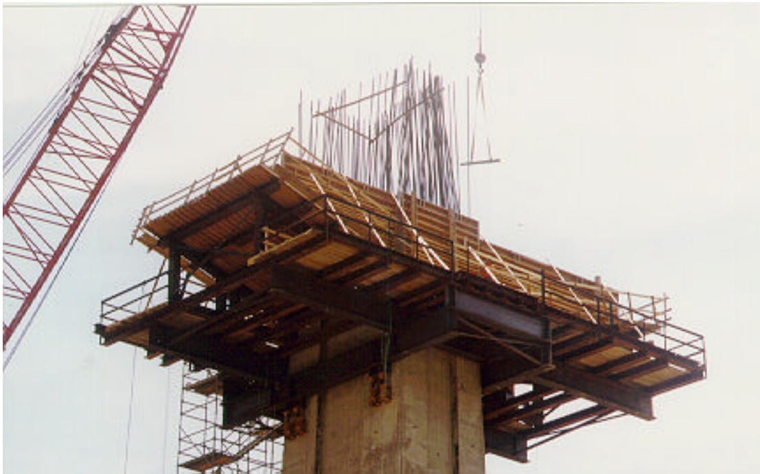
Figure 5-18: Pier 3 with Metal Falsework for Pier Table Erection
