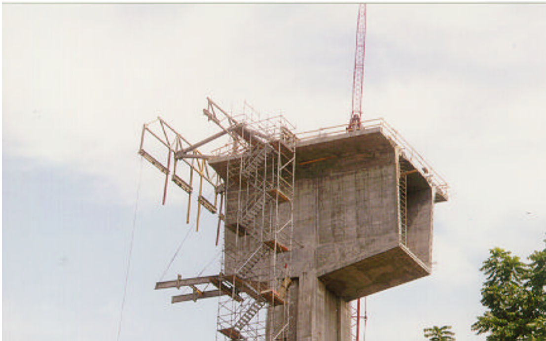
Figure 5-19: Pier Table 2 After Stripping from Formwork
