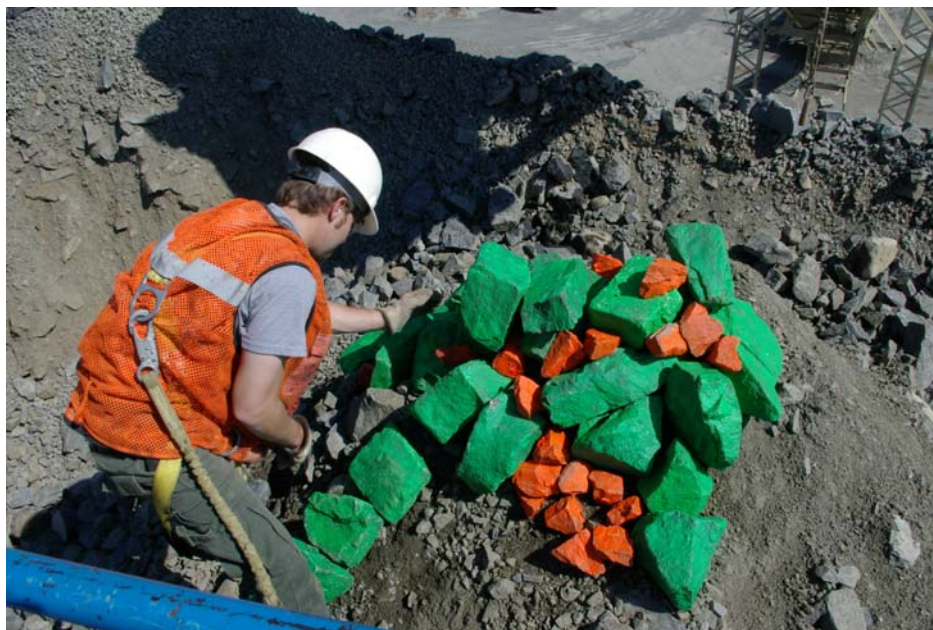
Figure 3.2 - Placement of rocks at peak of stockpile
