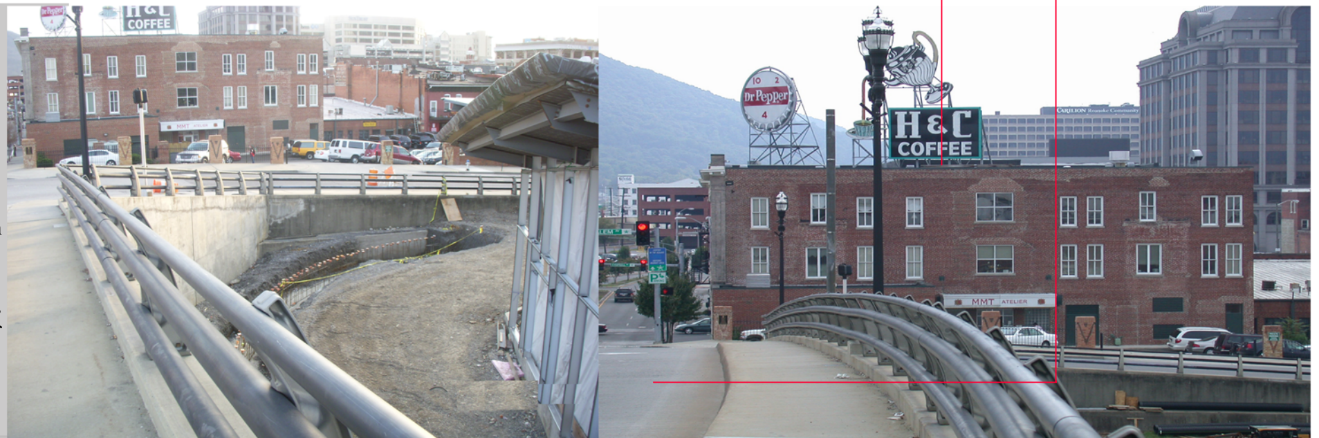
Corner Condition of the Site at the Intersection of Williamson Road and Salem Avenue
