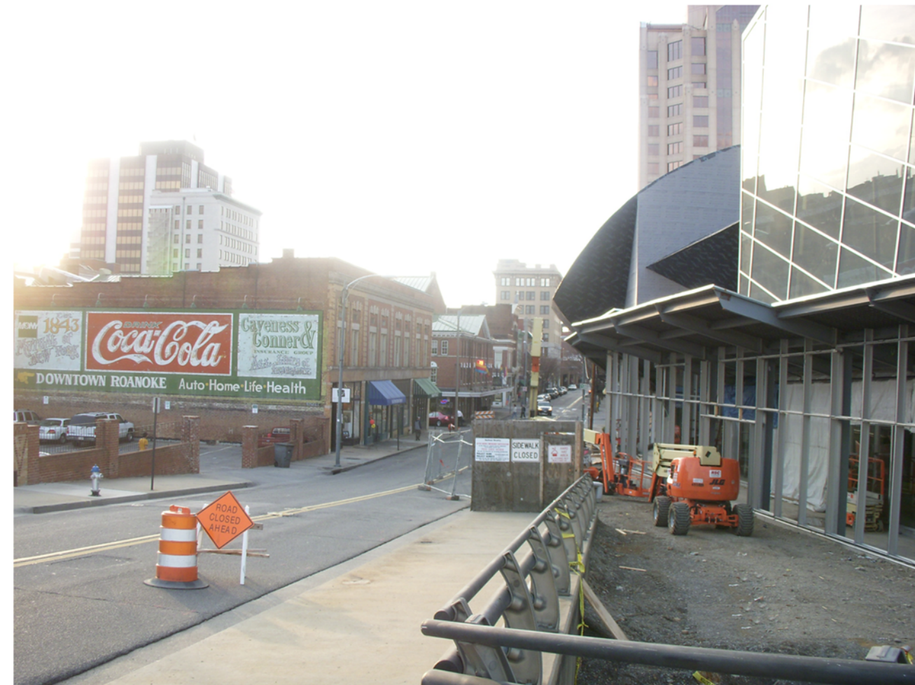
Existing Condition at the Site
