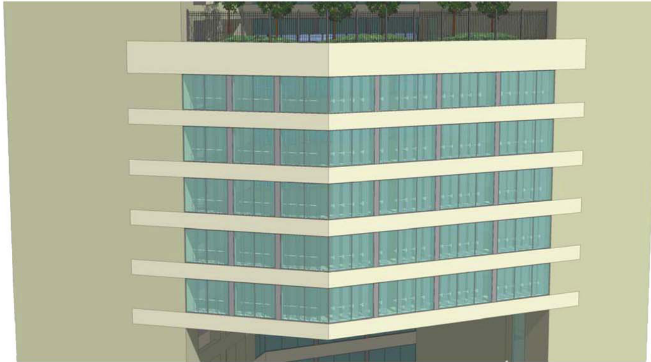
Fig 3.13 Exterior facade of office cluster
