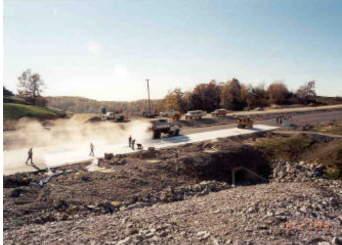
FIGURE 2 The asphalt distributor truck sprayed a tack coat on the road's surface.
