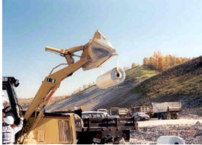
FIGURE 1 The membrane roll was lifted by the front-end loader.
