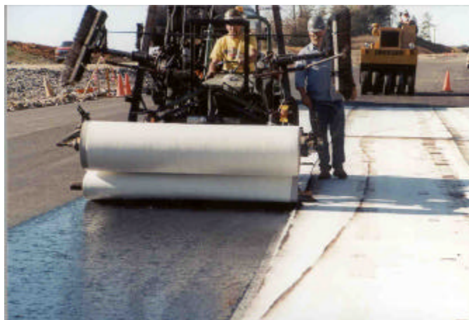
FIGURE 3 The installer unrolled the membrane on the heated tack coat.
