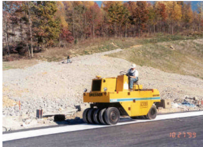
FIGURE 5 The compactor compacted the laid membrane.
