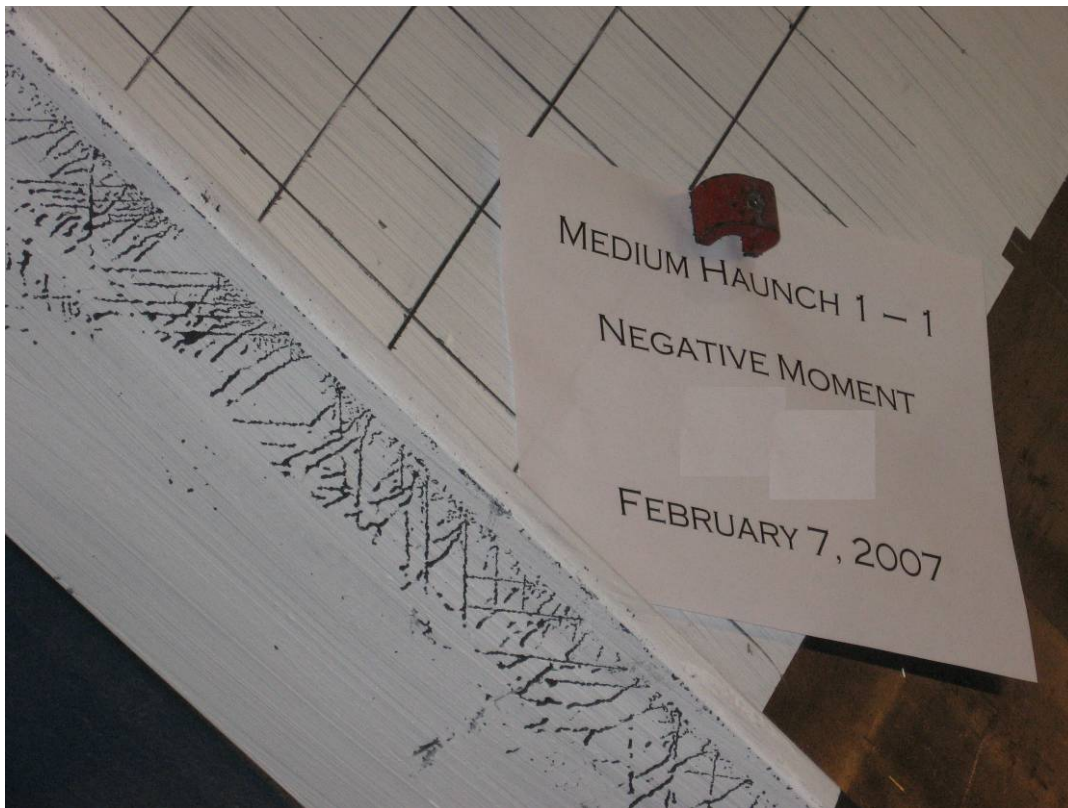
Figure F-1 MH 1 Rafter Compression Flange Yielding
