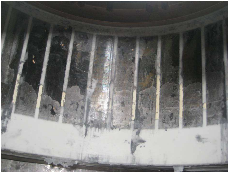
Figure 32 - Encapsulation Voids, Close Up - "Motor B"
